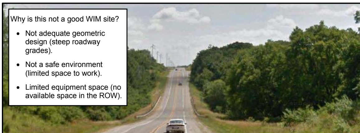
Figure 3.8: Poor WIM location
