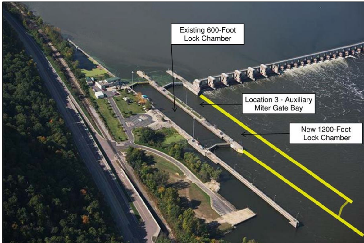
Figure 7: UMR Lock and Dam 22 – Auxiliary Miter Gate Bay with 1,200-foot Lock
