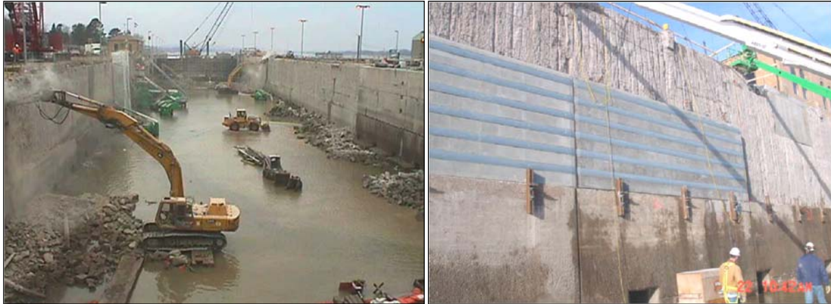
Figure 5: Major Rehabilitation Example – Chamber Concrete Rehabilitation
