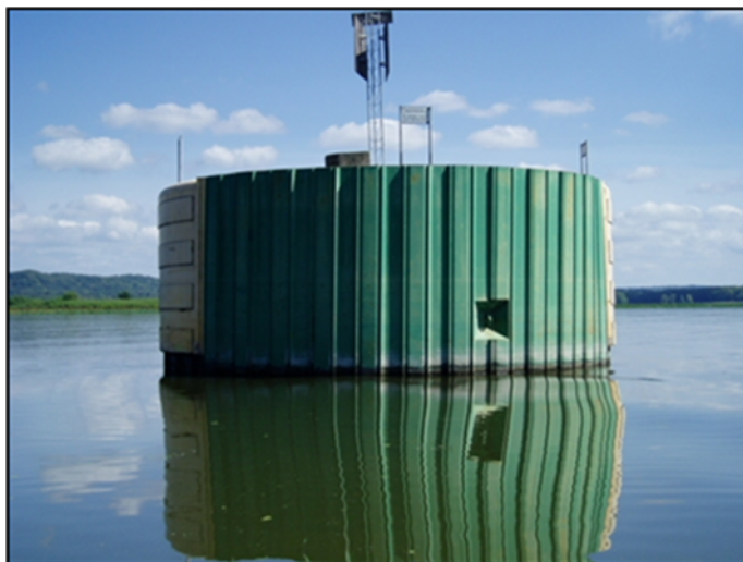
Figure 2: Typical Mooring Cell
