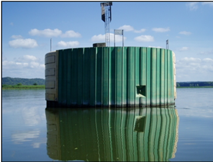
Figure 4: Typical Mooring Cell
