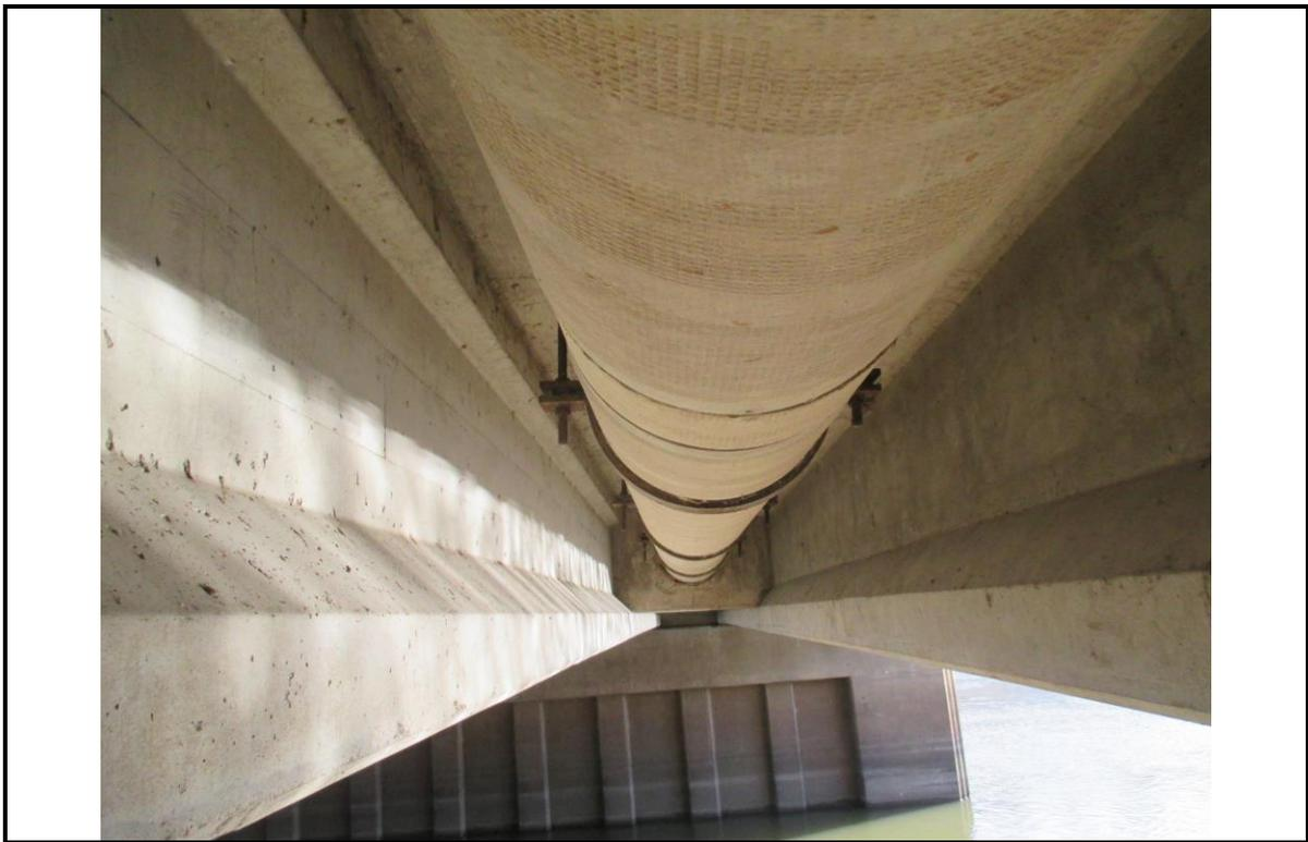
**Photo 2:** View of asbestos cement pipe under Park Road Bridge, looking east.
