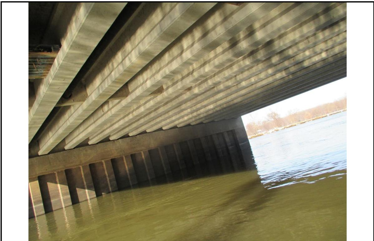
**Photo 6:** View of the girder layout under the east side of the Park Road Bridge.
