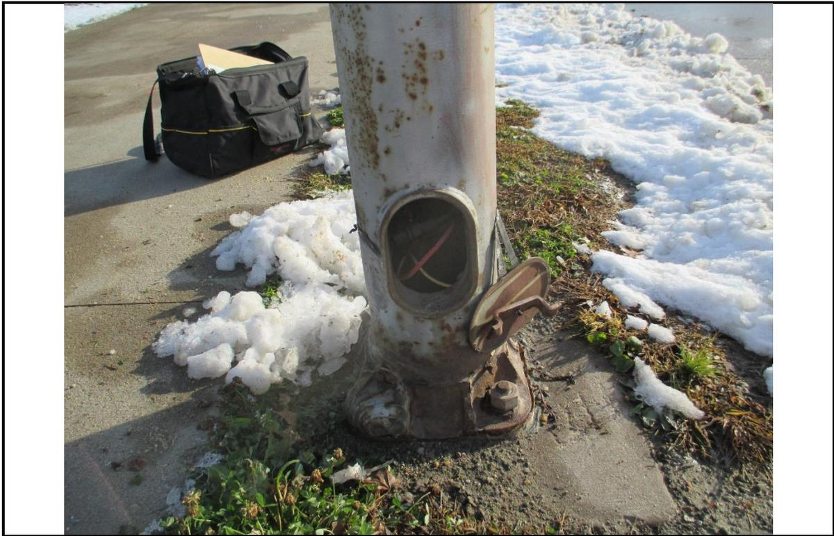
**Photo 7:** Photo showing chip location #1, and wiring inside of light post.
