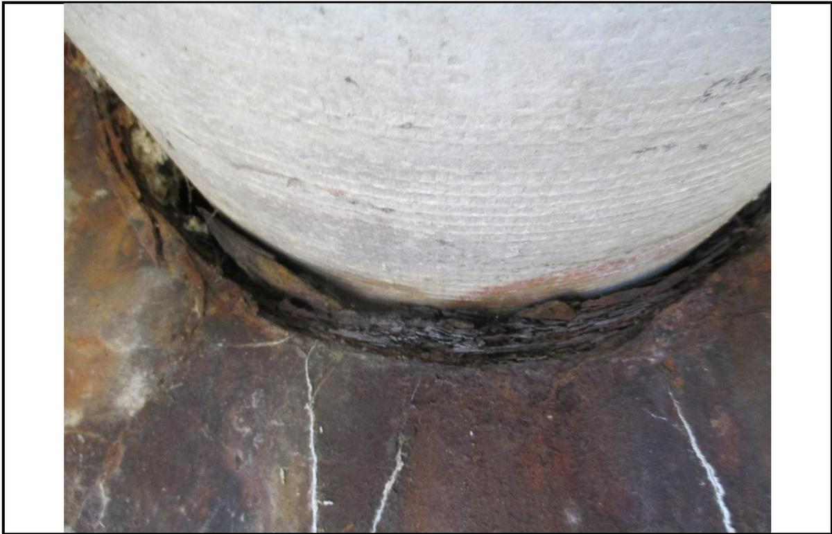
**Photo 3:** View of asbestos cement pipe as it enters the west abutment.
