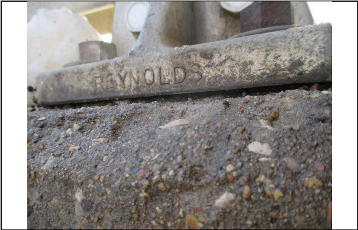
**Photo 5:** Photo showing trace asbestos under the guardrail post on Park Road Bridge.
