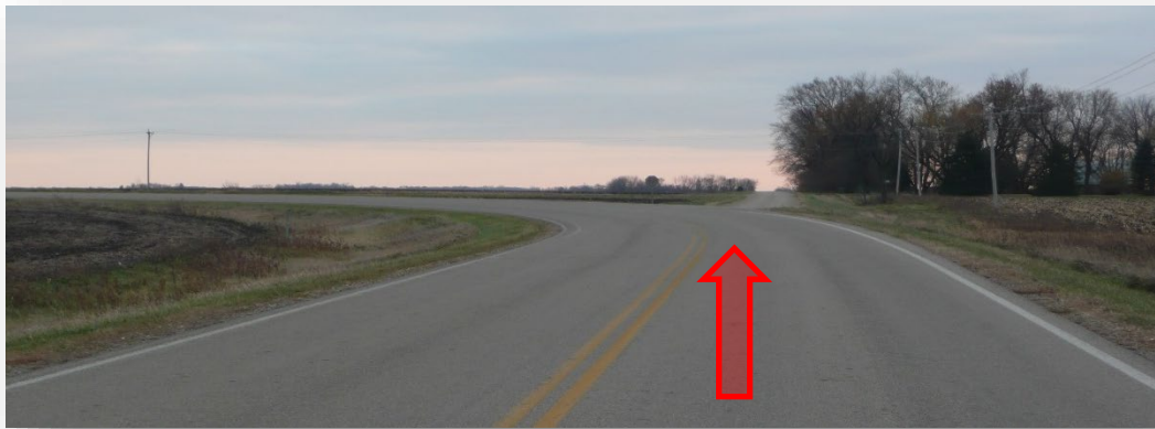
Figure 4. Example of a Visual Trap at a Horizontal Roadway Curve
