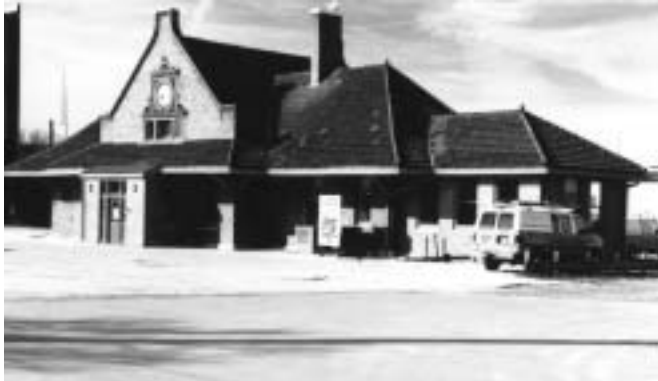
Davenport, Rock Island and Northwestern Railroad Depot
