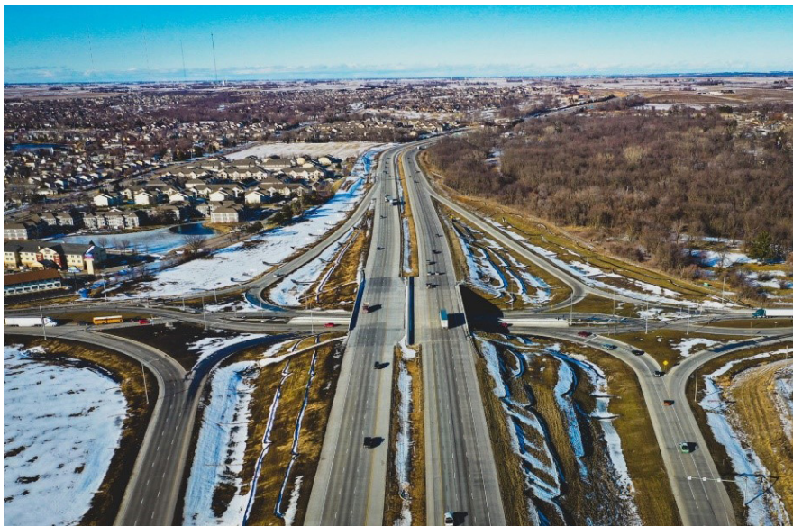
Diverging diamond interchange at I-35 and 1st Ave. in Ankeny. (Source: Iowa DOT)
