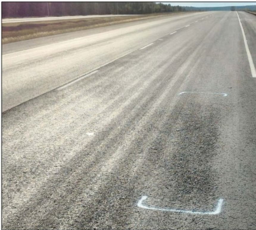
Photograph 8 – Moderate (bordering on Severe) Segregation
