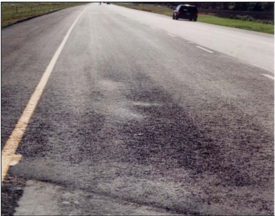
Photograph 10 - Severe Segregation
