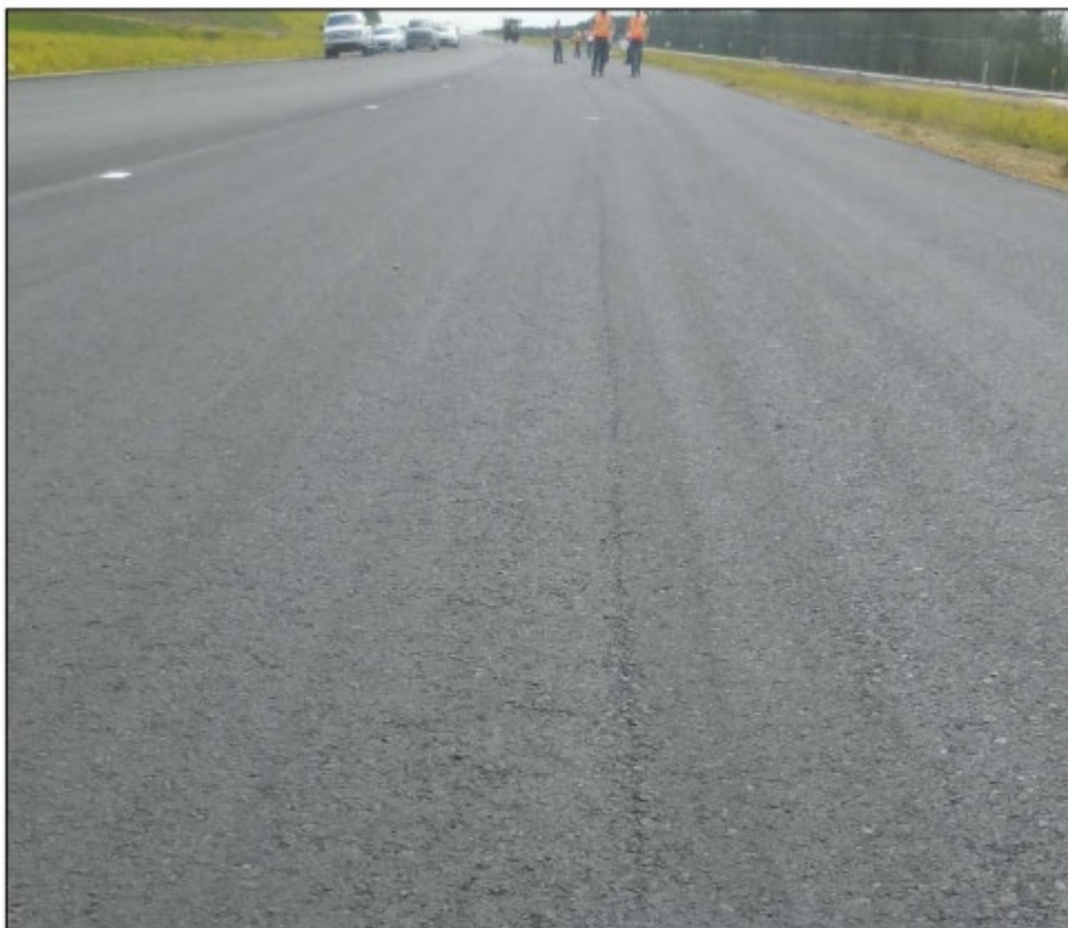
Photograph 13 - Centre-of-Paver Streak Classic case III in text
