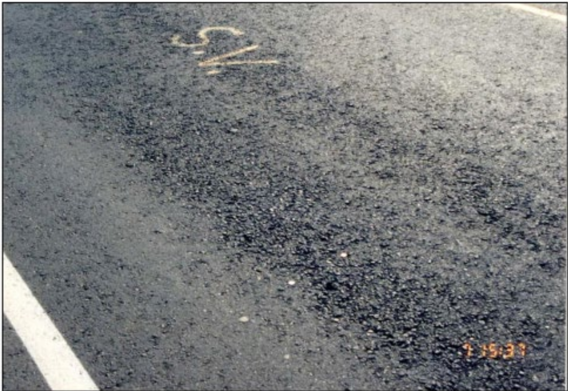
Photograph 11 - Severe Segregation
