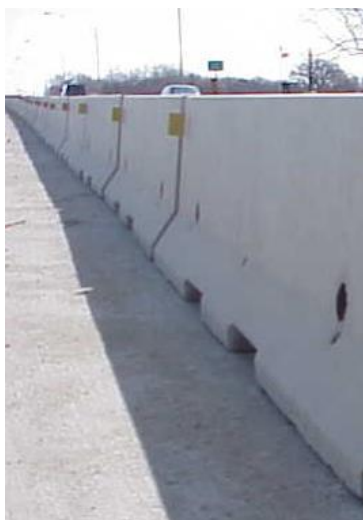
Figure 2: Temporary concrete barrier rail example.
