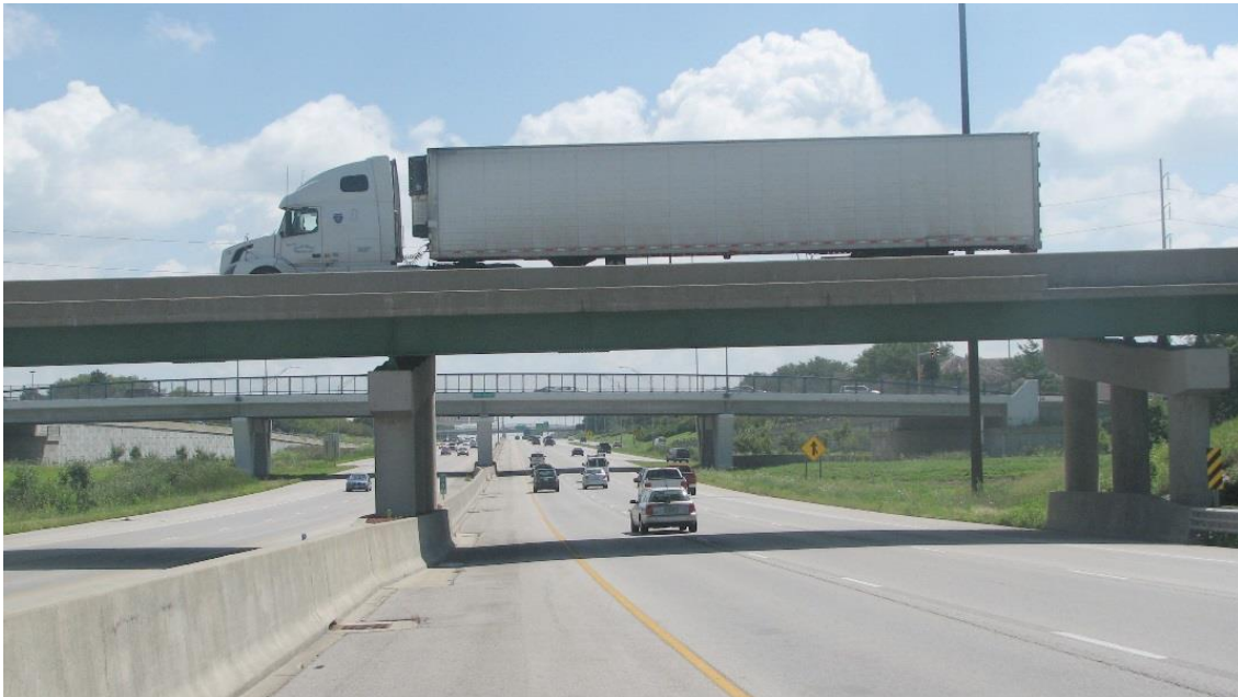
Figure 1: Permanent concrete barrier rail example.
