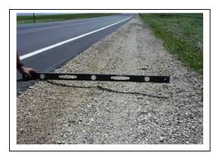
For resurfacing projects, additional granular material is added to existing shoulders to bring them up to the design cross section and eliminate drop-offs at the pavement edge. In some cases, earth fill is required prior to placing granular material.
