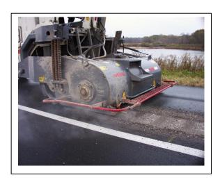
situations, utilizing a standard width, depth, and spacing. Differences lie in the distance offset from the painted edge line and the "skip" pattern specified for two-lane roadways and the outside shoulder of expressways. Grinding dimensions and alignment of the pattern should be randomly checked and adjusted, if necessary. Rumble strips are typically placed on mainline HMA shoulders only, with the pattern omitted at specified locations near intersections and ramps & loops.
