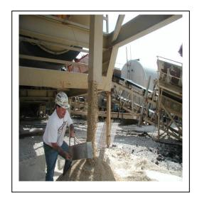
The inspector or monitor is typically required to direct and witness contractor sampling of other materials, such as aggregates and asphalt binder. The methods and procedures for sampling are given in applicable Materials IM's and are also taught in required lowa DOT certification courses. Minimum sampling frequencies are as stated in *IM 204*. All sampling done for project acceptance purposes must be directed and witnessed by the inspector or monitor.
