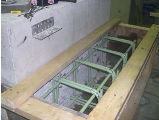
(a) Reinforcement inside a wooden form
