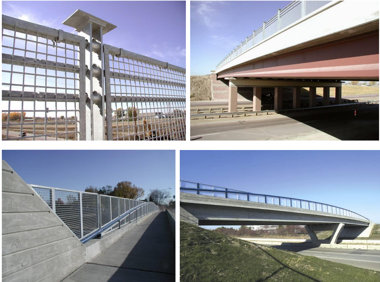
Figure 9.5.3.7-2. Bridges with complementary bolt-on aesthetic details
