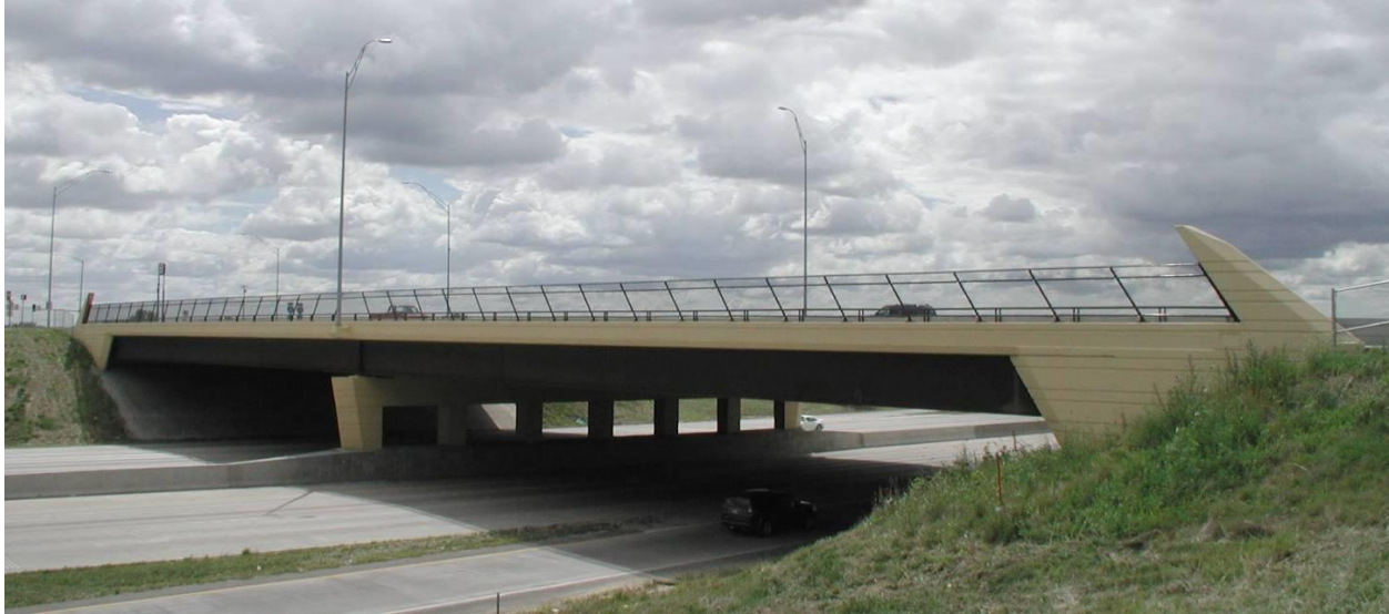
Figure 9.5.3.6. Bridge with sloping mask wall
