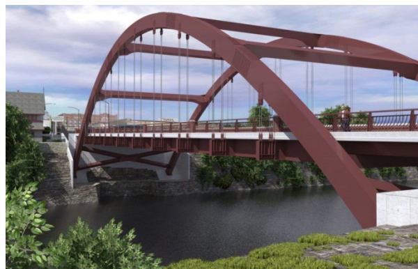
Figure 2.3.2-2 Replacement Steel Arch Bridge
