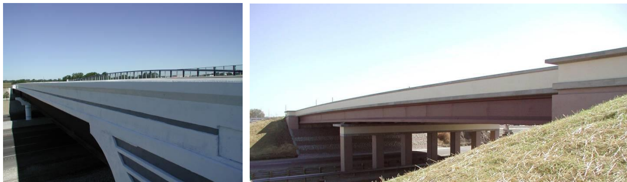
Figure 9.5.3.1. Bridges with long, slender appearance
