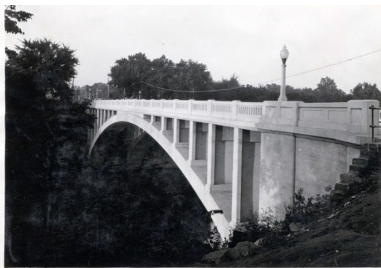
Figure 2.3.2-1 Original Concrete Arch Bridge
