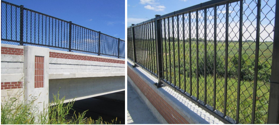
Figure 5.8.1.2.5-2. Example Welded Picket Railing with Chain Link Mesh (project shown is NHSX-100-1(93)—3H-57, Linn. Co. Design No. 915)
