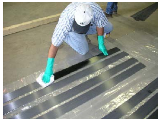
(b) Cleaning CFRP plates
