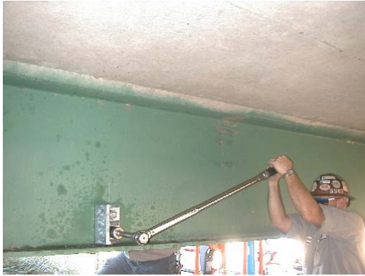
(a) Installation of anchorage assembly
