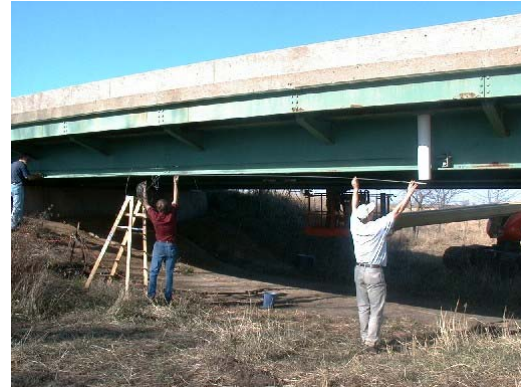
(b) Placement of CFRP rod
