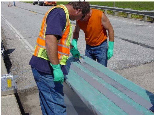
(c) Epoxy application on CFRP plates
