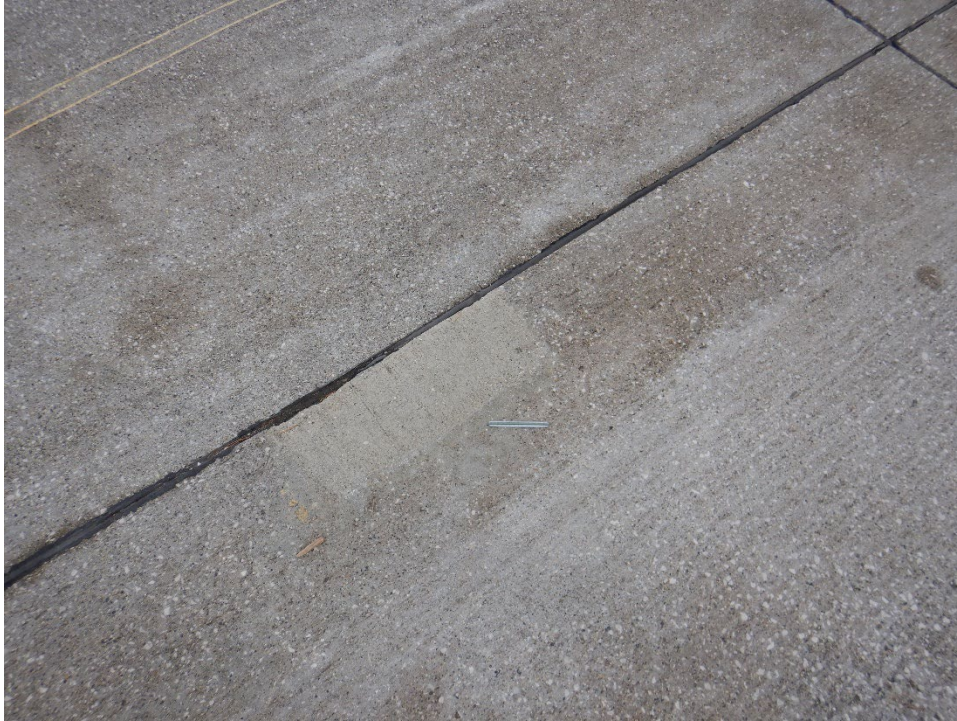
A01WC-02. Small Patching (Sample Unit No. 04).
