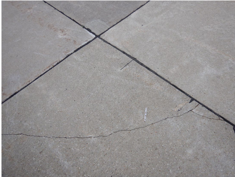
TH01WV-02. Corner Break (Sample Unit No. 01).
