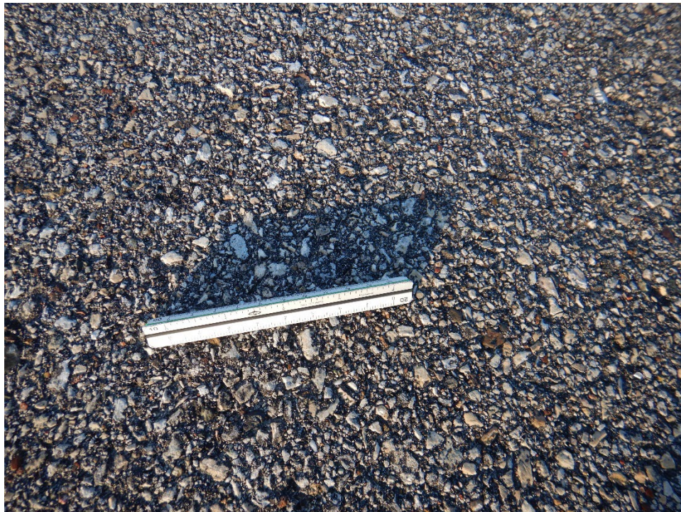
A01WK-01. Weathering (Sample Unit No. 04).
