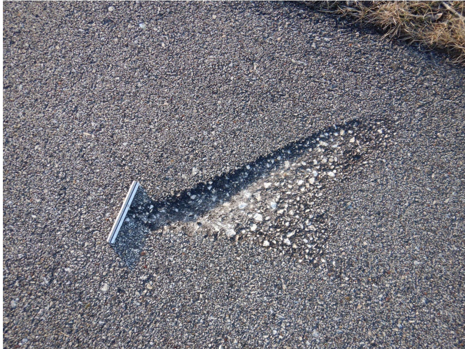
A01WK-01. Raveling (Sample Unit No. 04).
