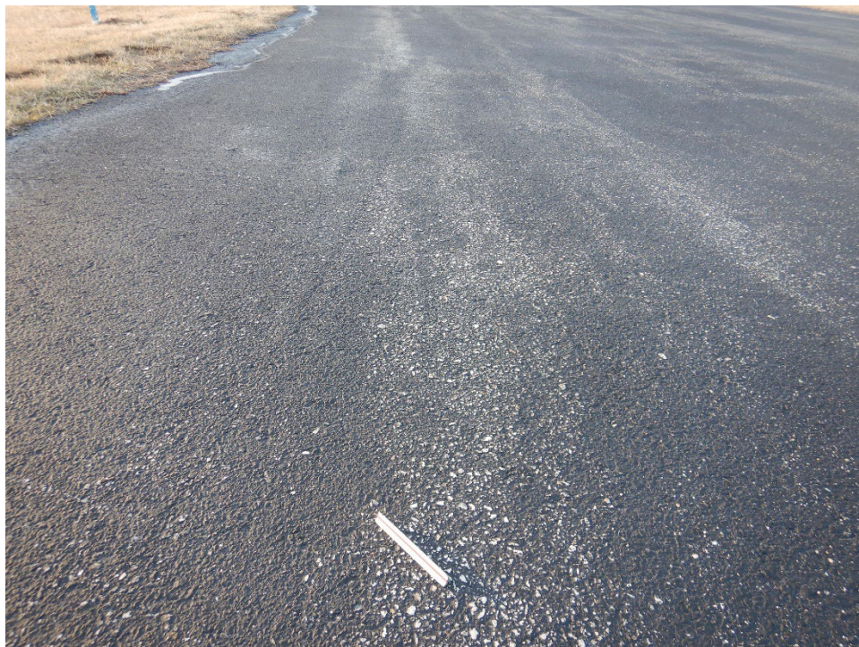
T02WK-01. Weathering (Sample Unit No. 01).
