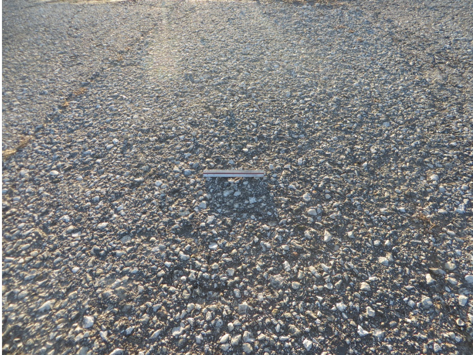
A01WK-01. Raveling (Sample Unit No. 04).
