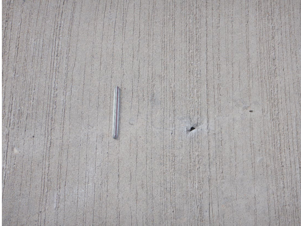
TBWA-03. ASR (Additional Sample Unit No. 10).
