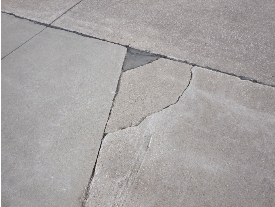
A01WA-06. Corner Break (Sample Unit No. 01).
