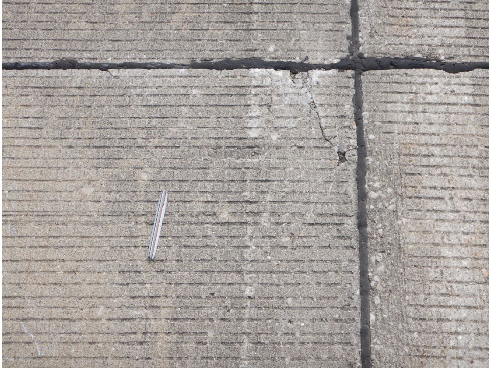
R18WA-01. ASR (Sample Unit No. 12).
