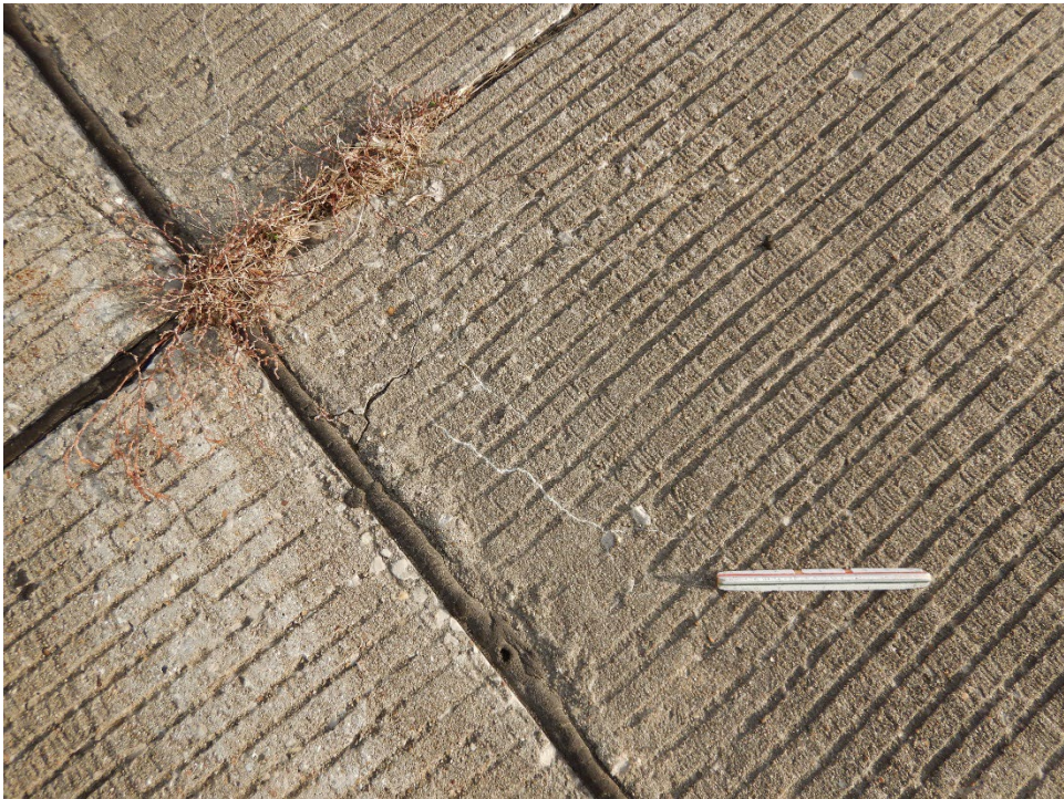
R18WA-01. ASR (Additional Sample Unit No. 08).
