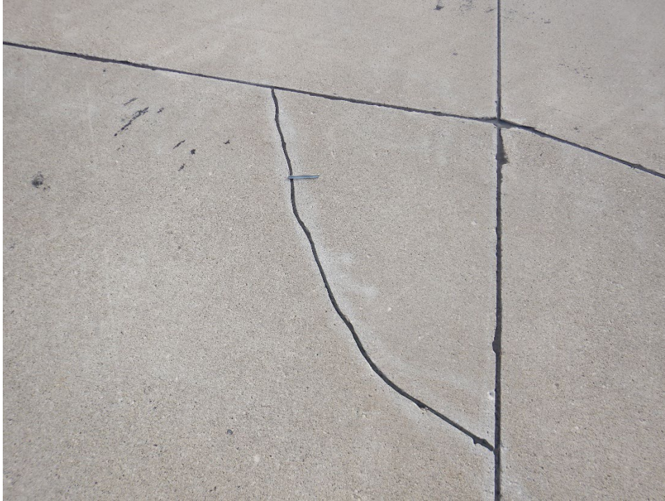
TASP-01. Corner Break (Additional Sample Unit No. 01).
