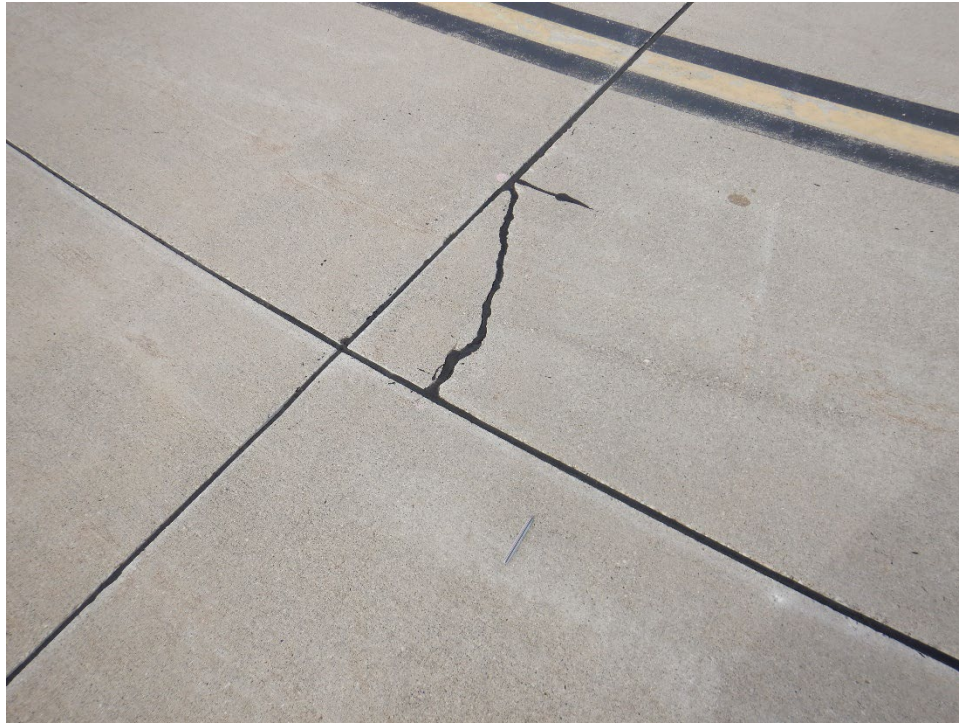
TDSP-01. Corner Break (Sample Unit No. 20).
