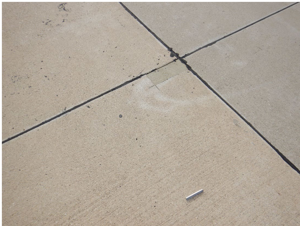
A01SP-05. Small Patching (Sample Unit No. 04).
