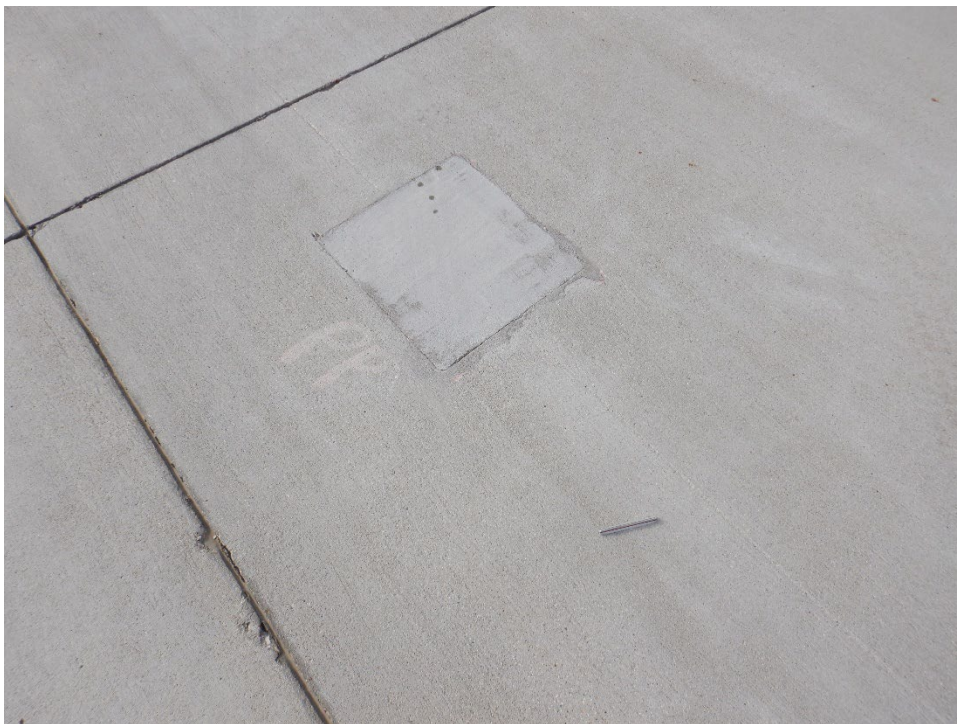
A01SP-01. Small Patching (Sample Unit No. 02).
