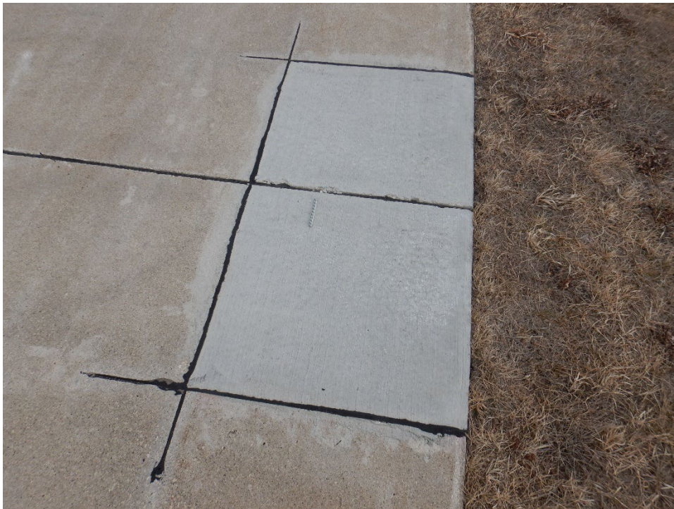
TASP-02. Small Patching (Additional Sample Unit No. 03).
