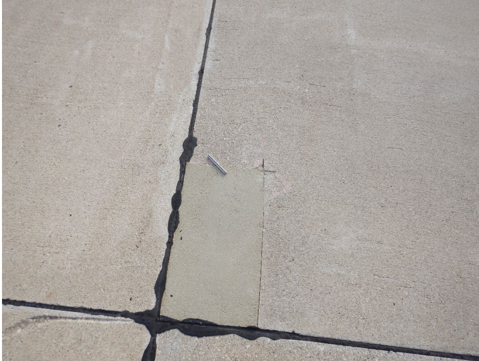
A01SP-04. Small Patching (Sample Unit No. 09).
