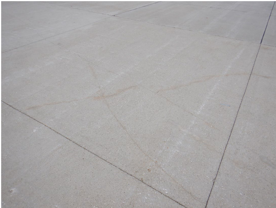
A01SX-03. Shattered Slab (Sample Unit No. 01).
