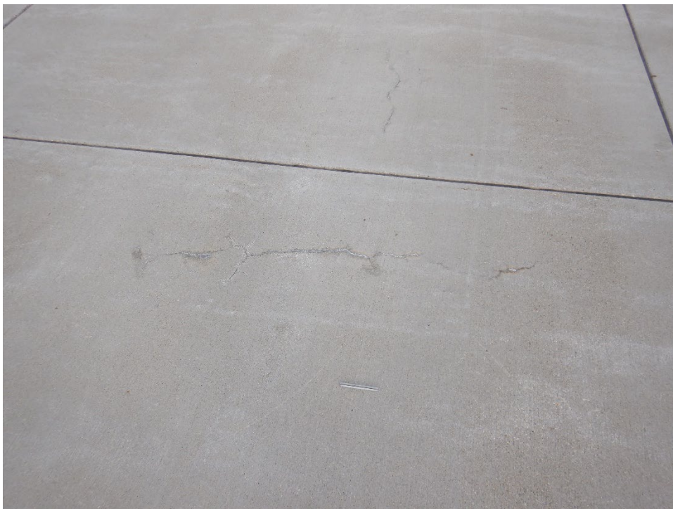
A01SX-01. ASR (Additional Sample Unit No. 41) (1).
