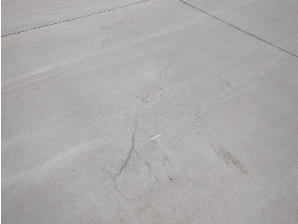
A01SX-01. ASR (Additional Sample Unit No. 41) (2).
