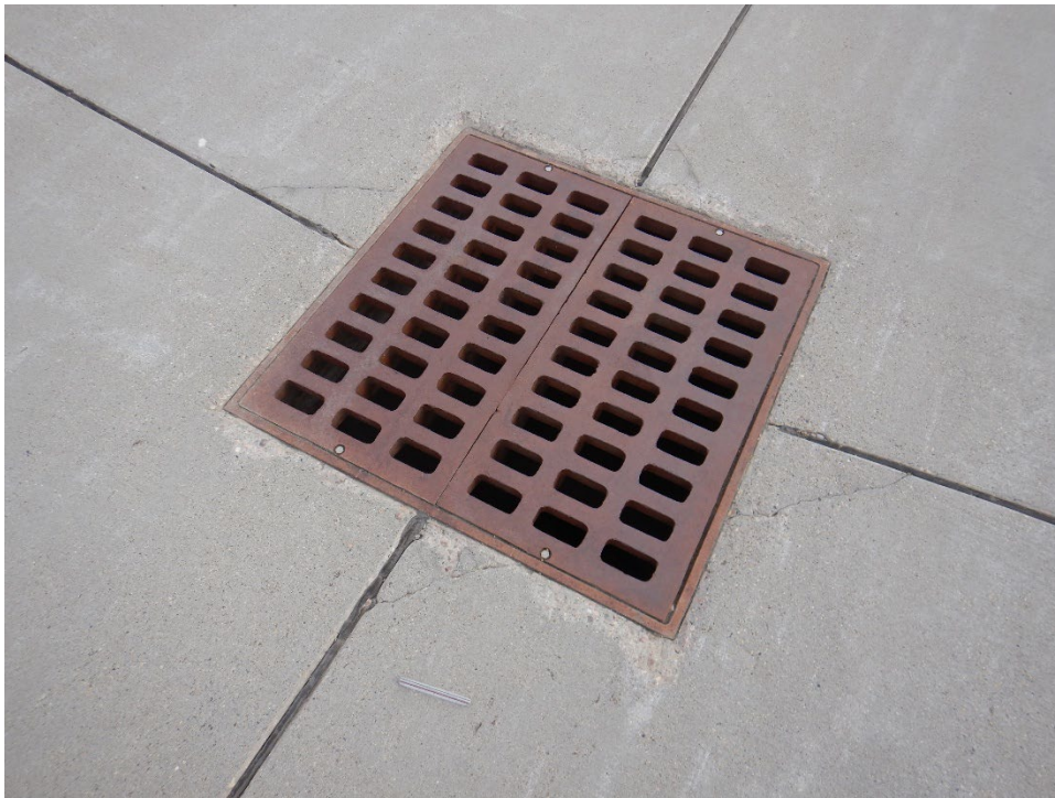
A01SX-01. Corner Spalling (Sample Unit No. 47).
