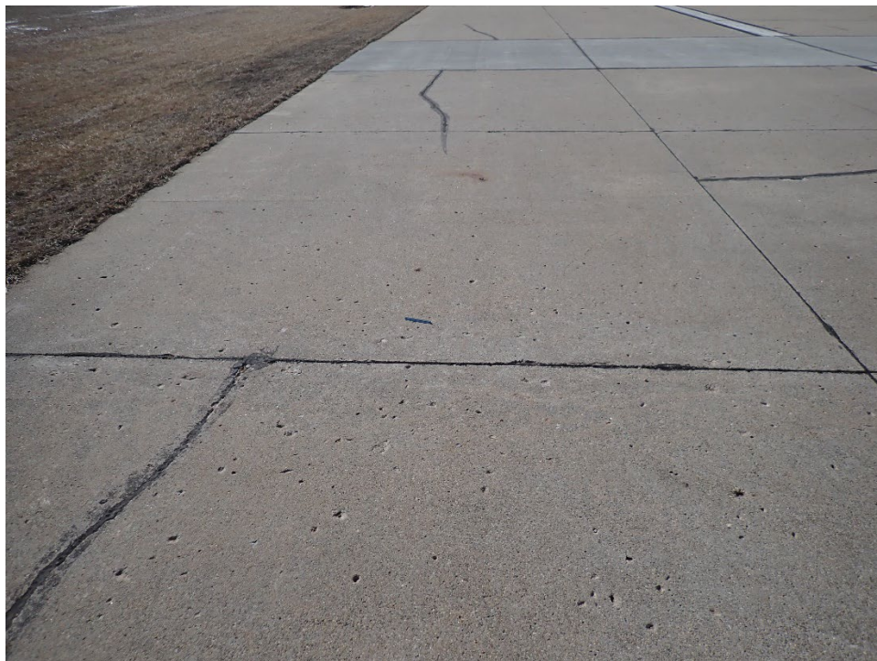
R17IS-01. Popouts (Sample Unit No. 32).
