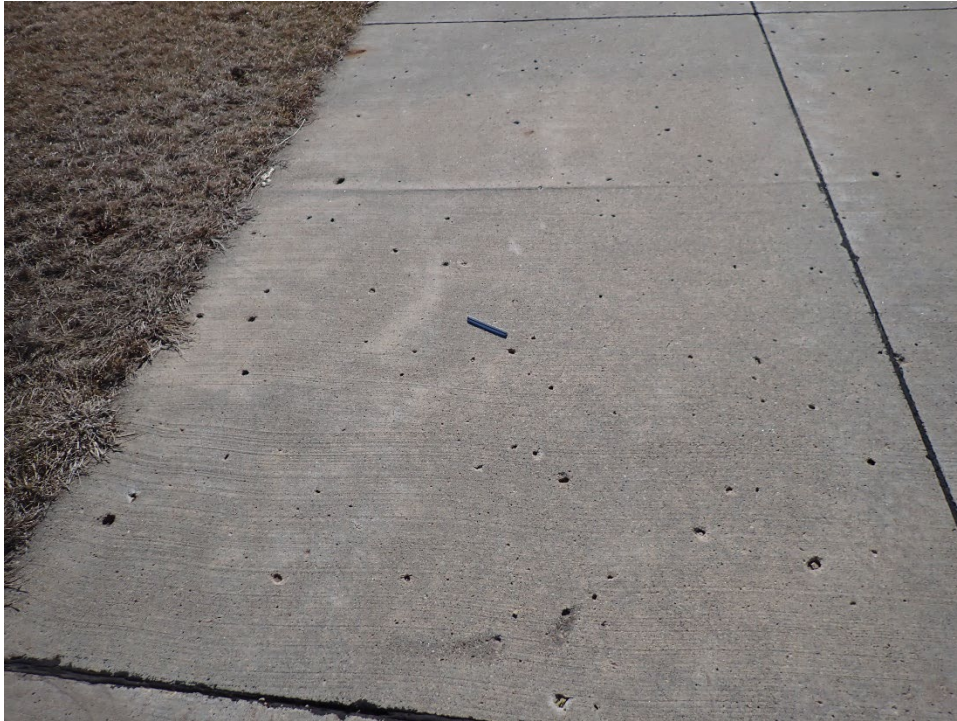
T03IS-03. Popouts (Sample Unit No. 01).
