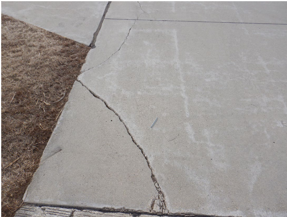
A01SD-04. Corner Break (Sample Unit No. 05).
