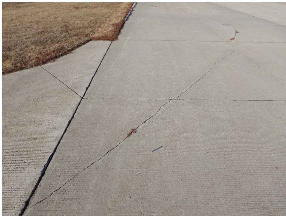
A01SD-02. Corner Break (Sample Unit No. 03).
