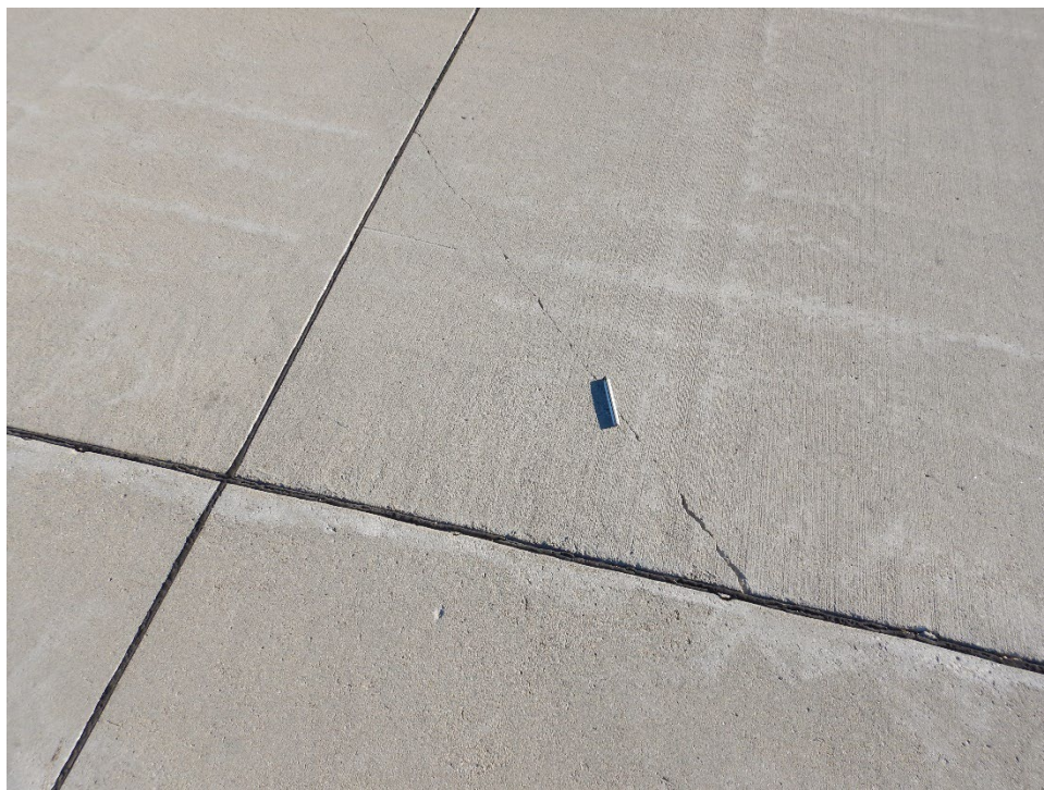
A01SD-04. Corner Break (Sample Unit No. 02).
