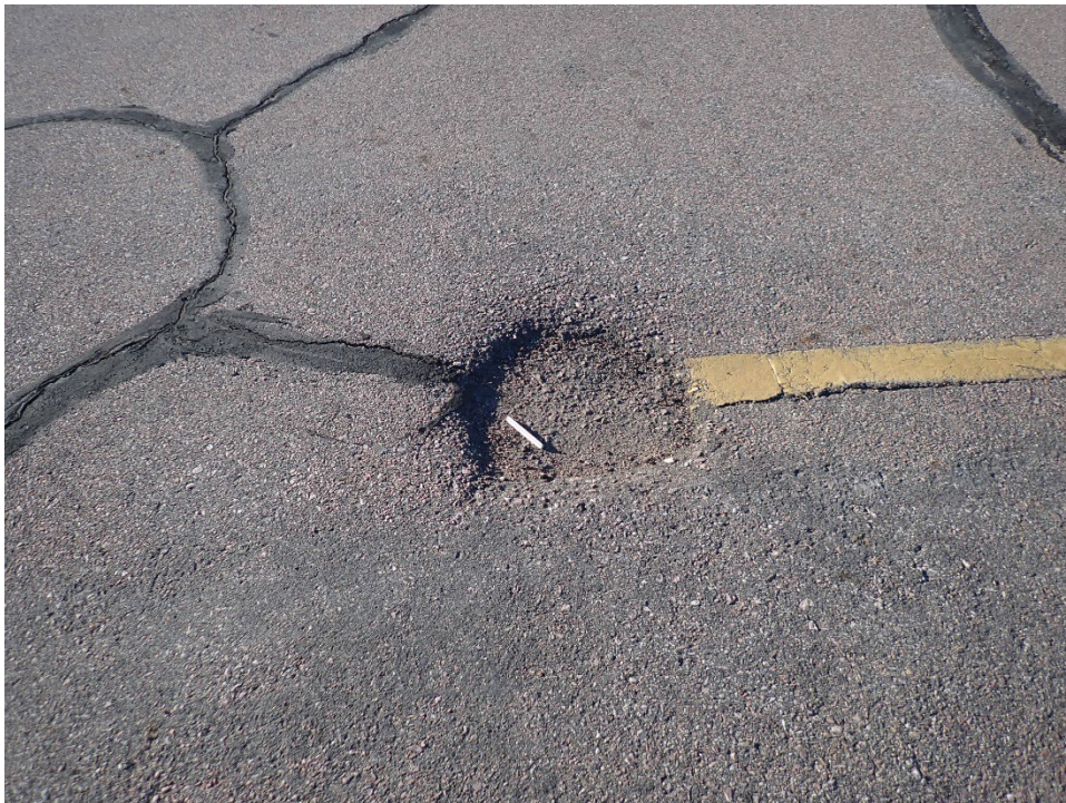
A01RR-01. Raveling (Sample Unit No. 03) (2).
