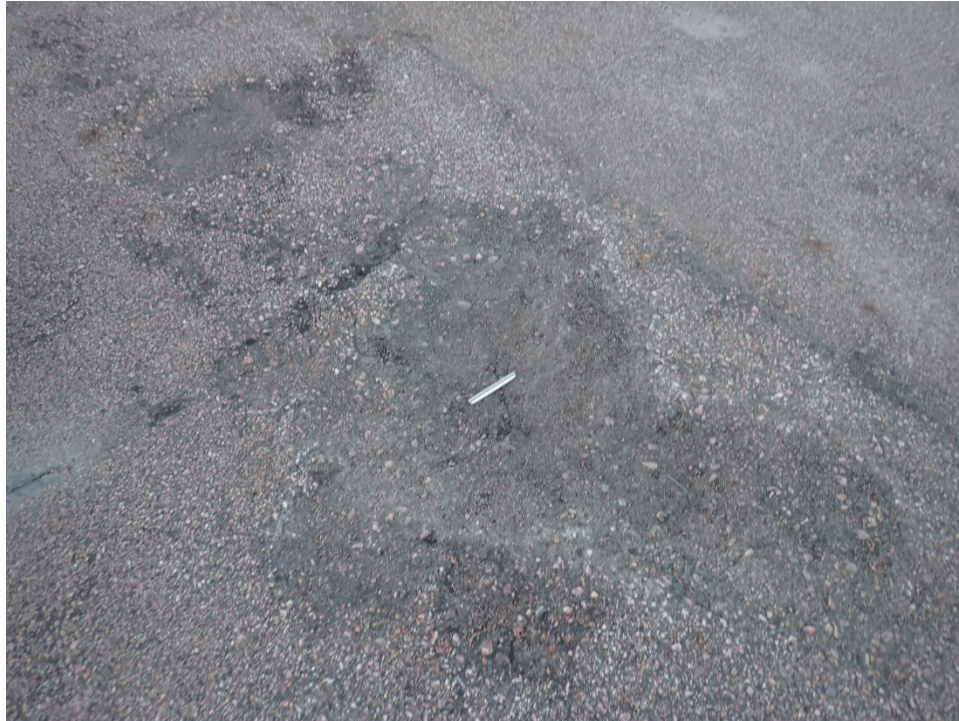
R16RR-01. Raveling (Sample Unit No. 01).
