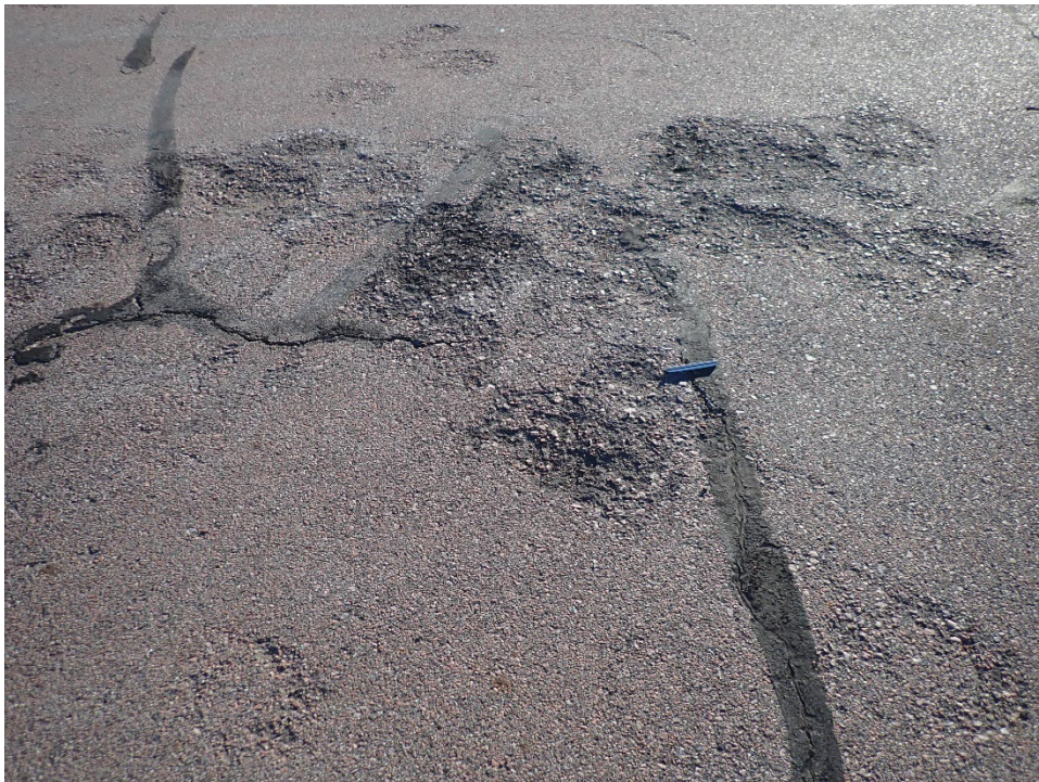
R16RR-03. Raveling (Sample Unit No. 03).
