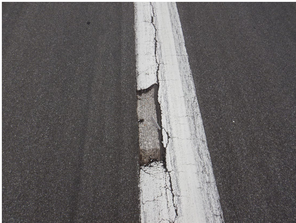
R12PO-01. Raveling (Sample Unit No. 28).
