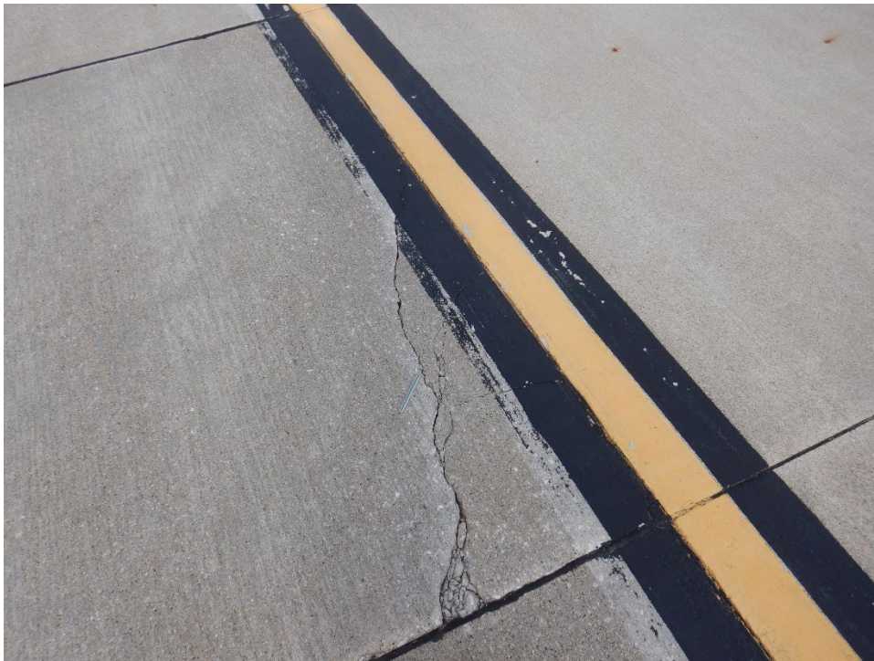
T02PO-01. Corner Break (Sample Unit No. 01).
