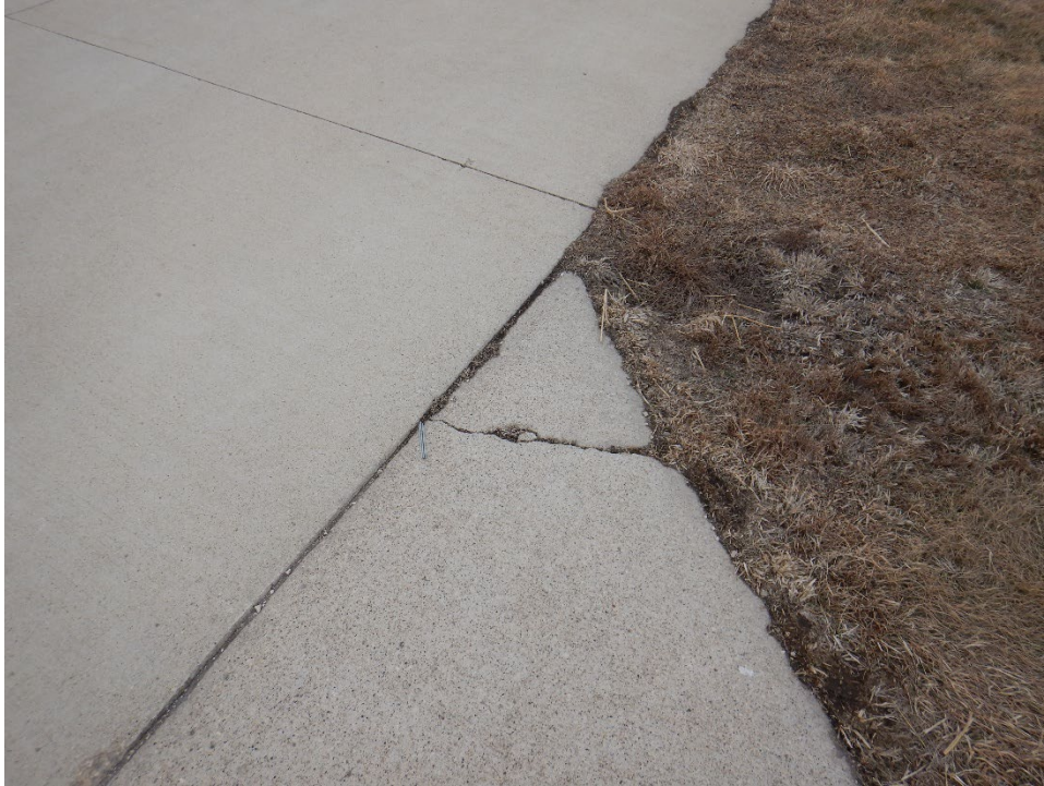
TH01PO-02. Corner Break (Sample Unit No. 01).
