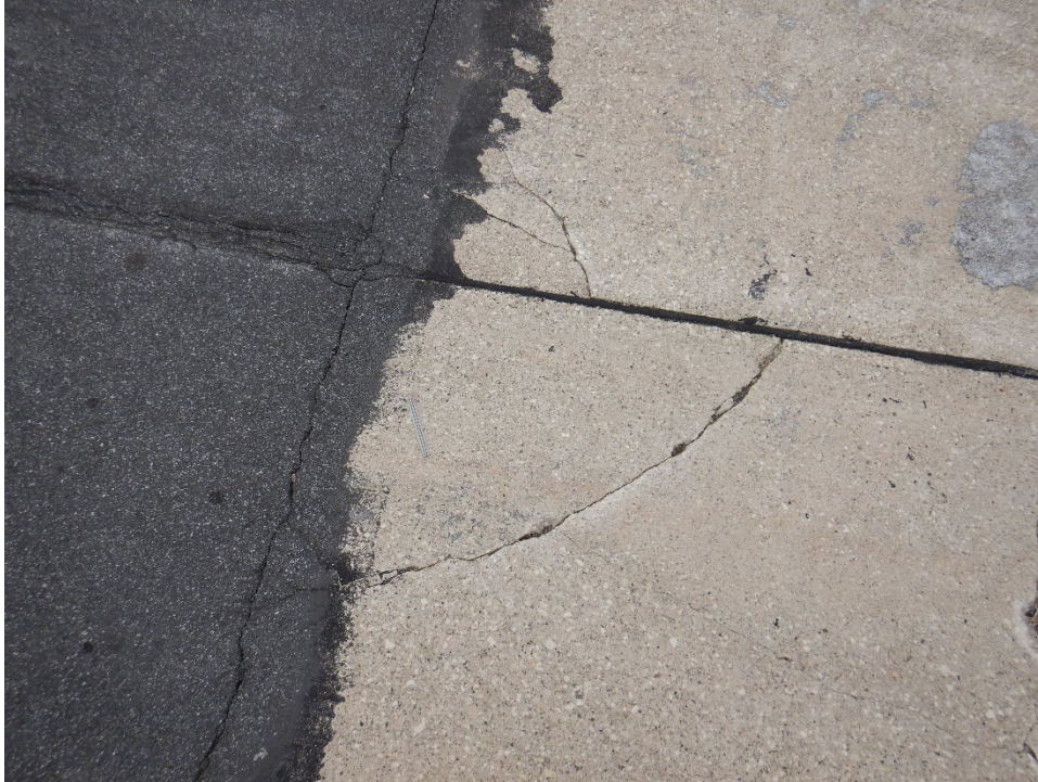
T01PO-01. Corner Break (Sample Unit No. 01).
