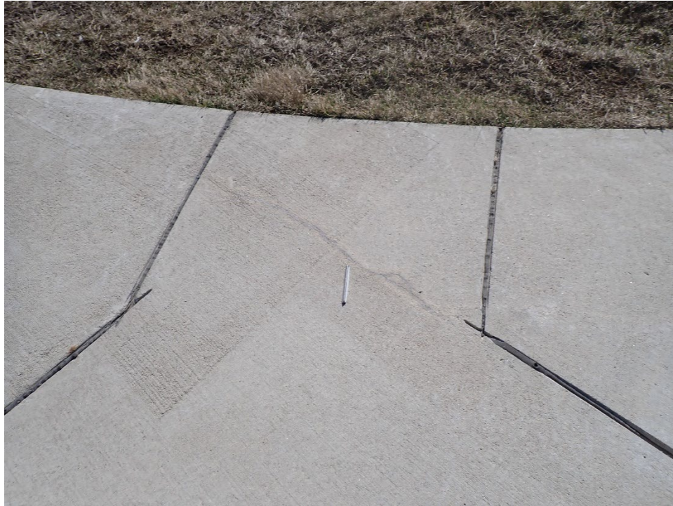
T01PE-02. ASR (Sample Unit No. 01).
