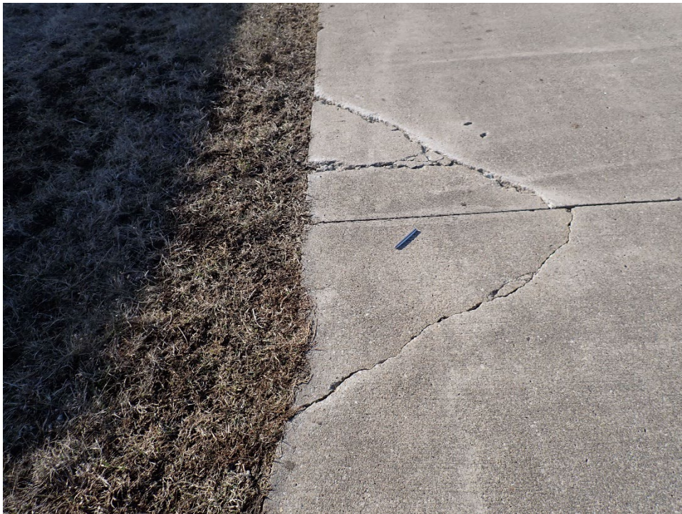
TH01PE-01. Corner Break (Sample Unit No. 09).
