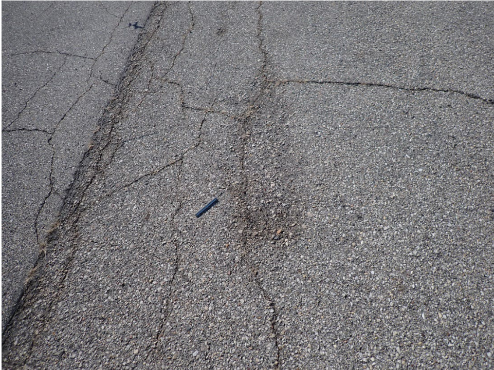
T011Y-02. Raveling (Sample Unit No. 01).
