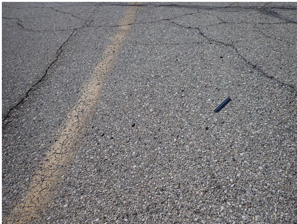
T011Y-01. Raveling (Sample Unit No. 01).
