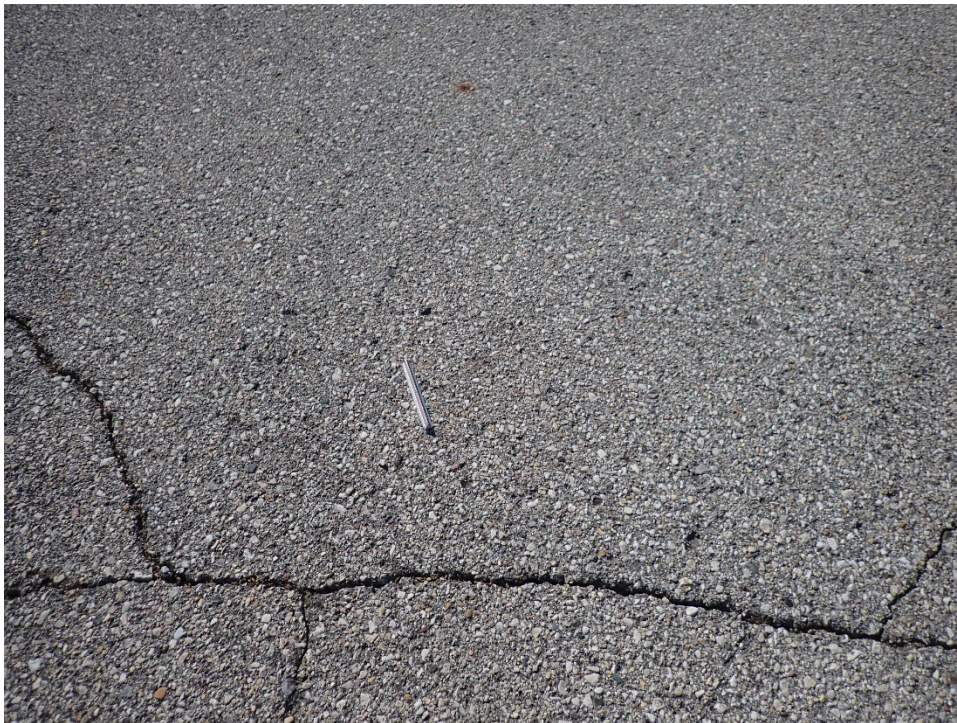
T011Y-03. Raveling (Sample Unit No. 01).
