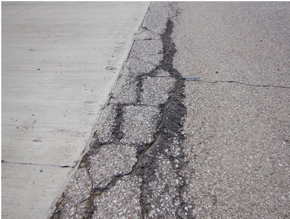
TBOT-06. Shoving (Sample Unit No. 02).
