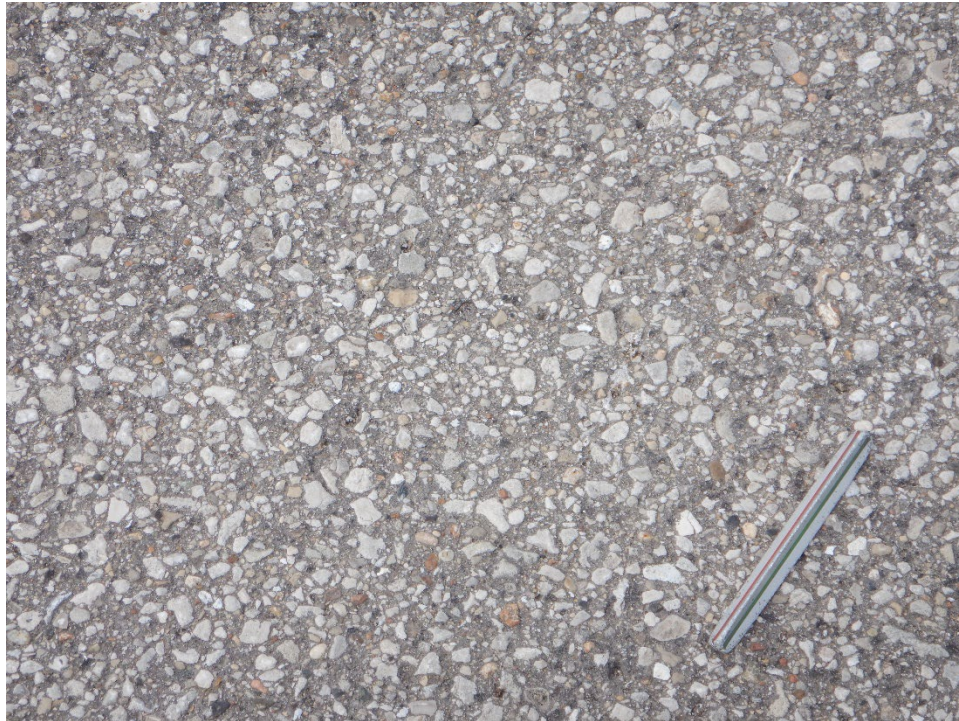
A01OT-02. Weathering (Sample Unit No. 02).
