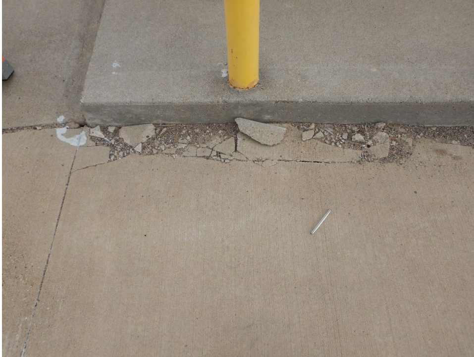
A01OT-06. Blow-Up (Sample Unit No. 12).
