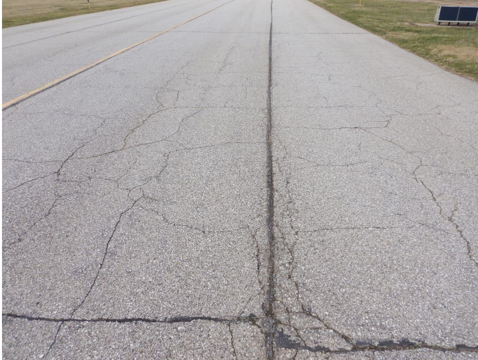
TAOT-06. Block Cracking (Sample Unit No. 06).
