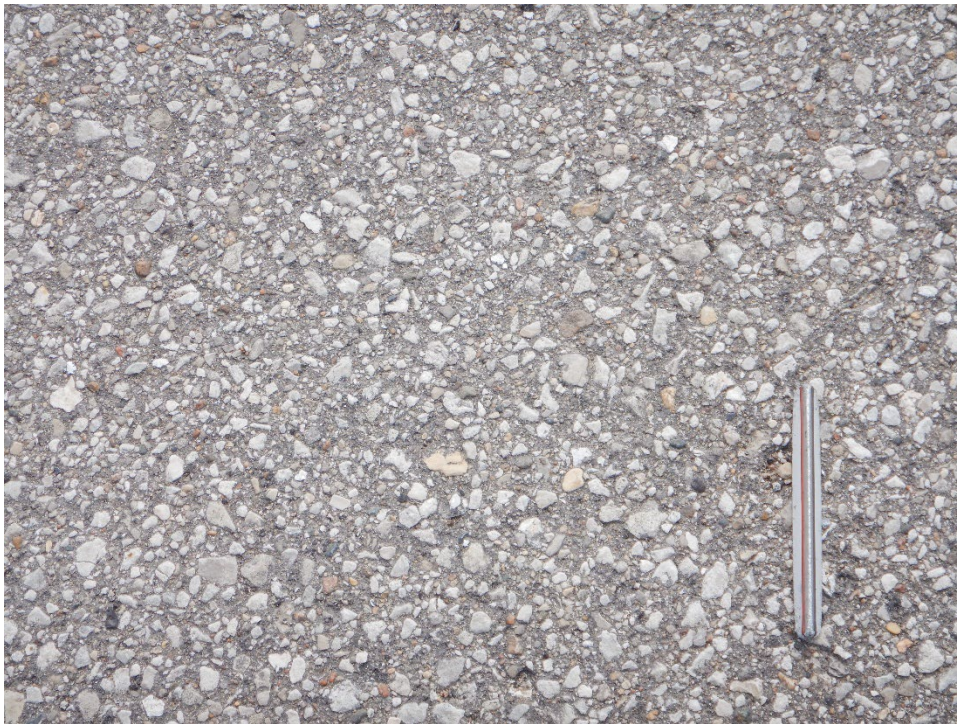
A01OT-01. Weathering (Sample Unit No. 02).
