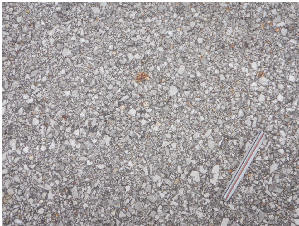
TAOT-01. Weathering (Sample Unit No. 11).
