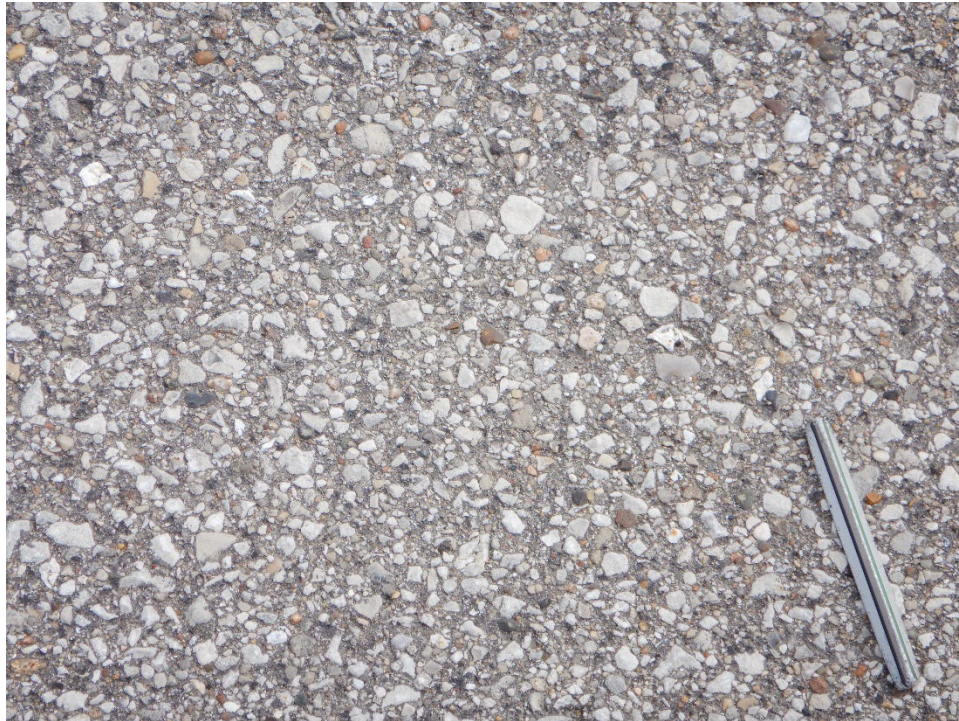
A02OT-01. Weathering (Sample Unit No. 02).
