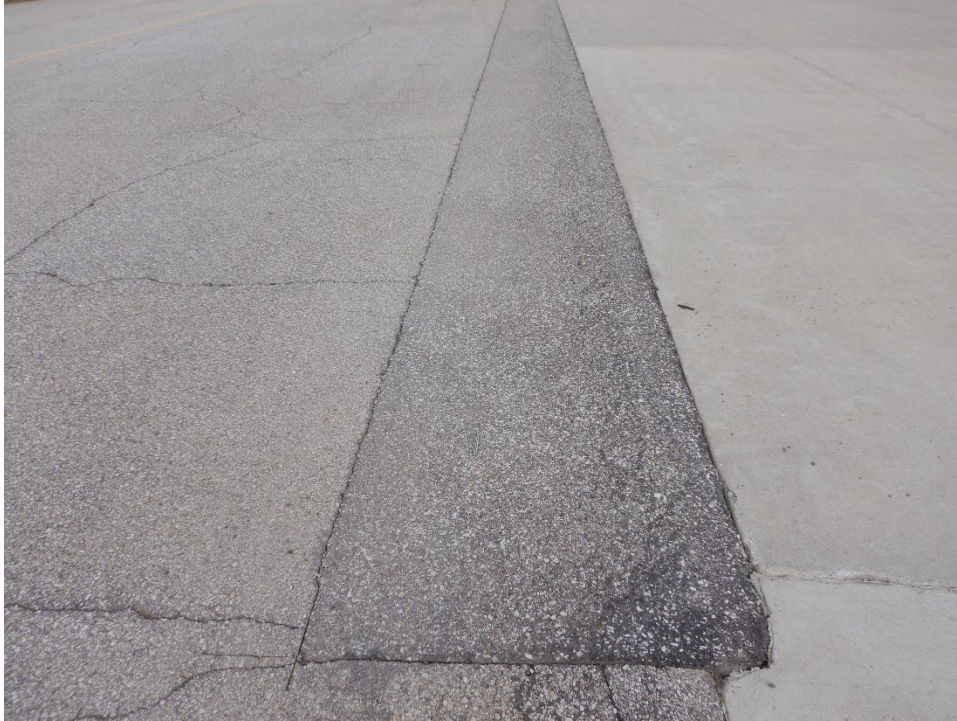
TBOT-06. Patching (Sample Unit No. 01).
