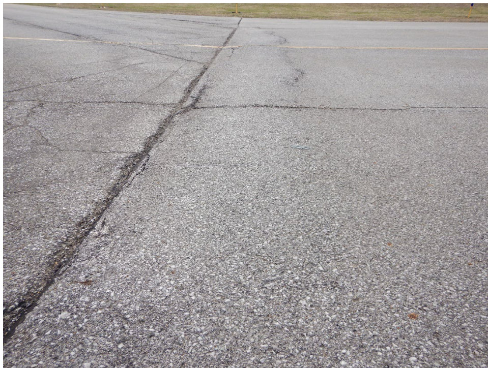
TBOT-02. Swelling (Sample Unit No. 02).
