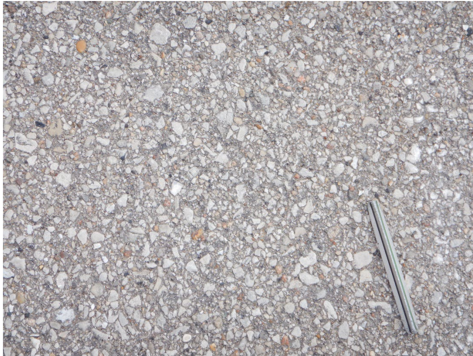
A01OT-05. Weathering (Sample Unit No. 02).
