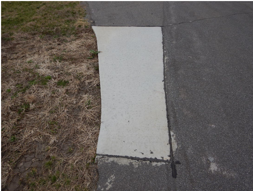
TCOT-01. Patching (Sample Unit No. 03).
