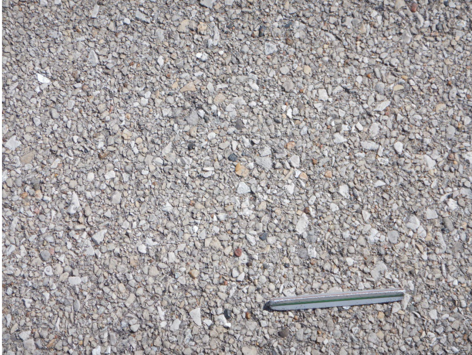
A02OT-04. Weathering (Sample Unit No. 01).
