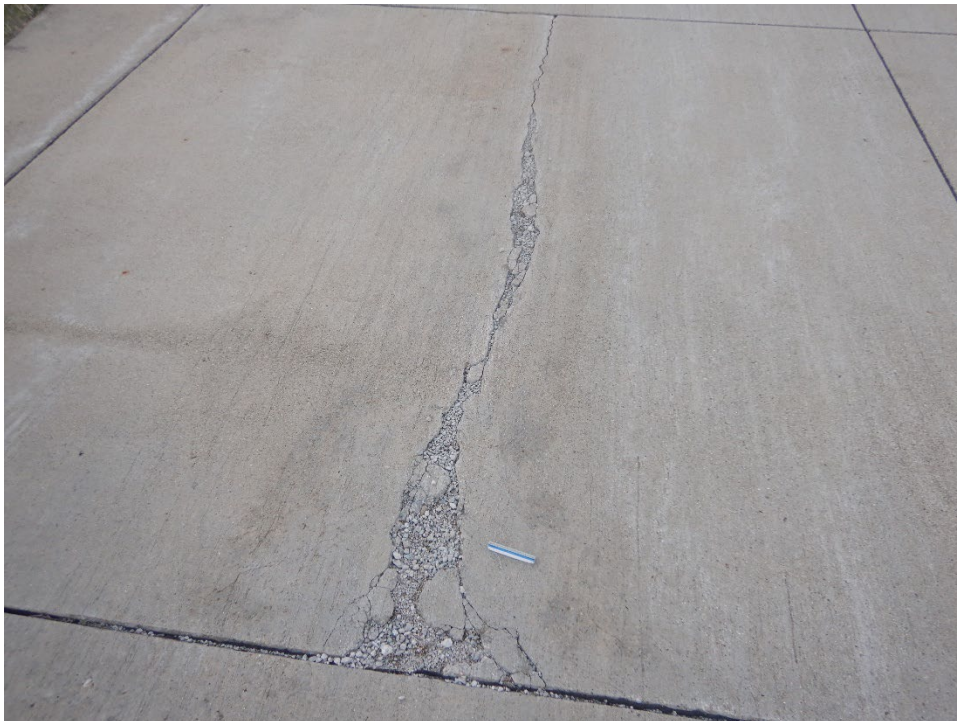
T05OK-03. ASR (Additional Sample Unit No. 01).
