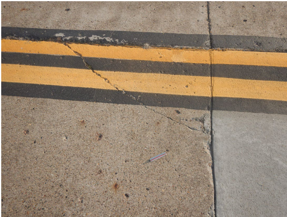
T01OK-03. Corner Break (Sample Unit No. 02).
