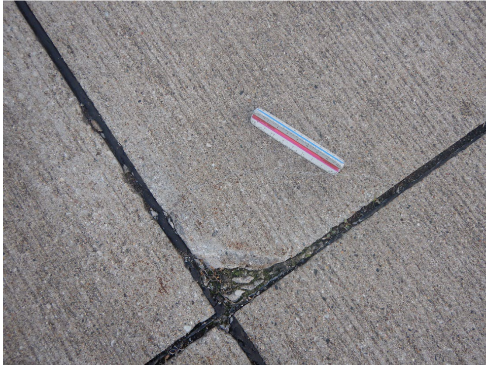
R13OK-01. ASR (Additional Sample Unit No. 66).
