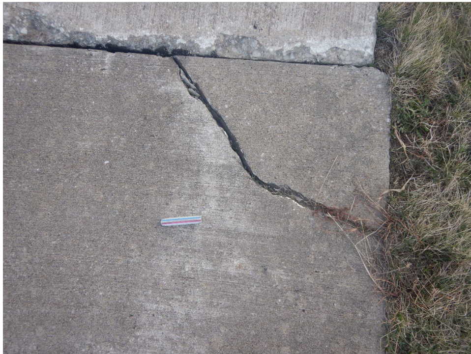
R13OK-01. Corner Break (Sample Unit No. 01).
