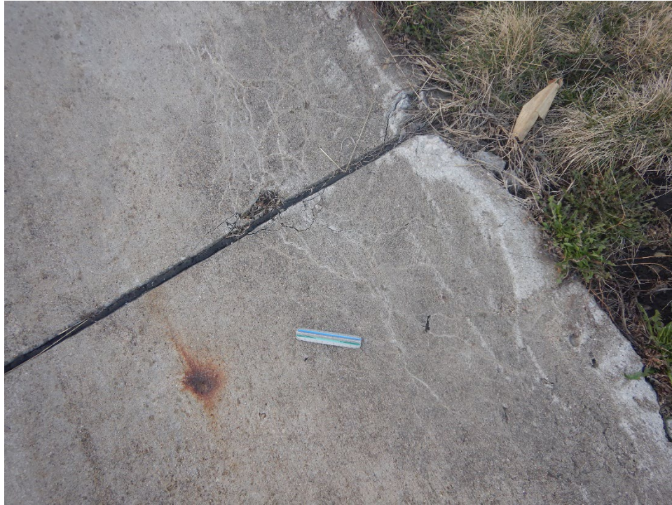
T05OK-03. ASR (Sample Unit No. 12).
