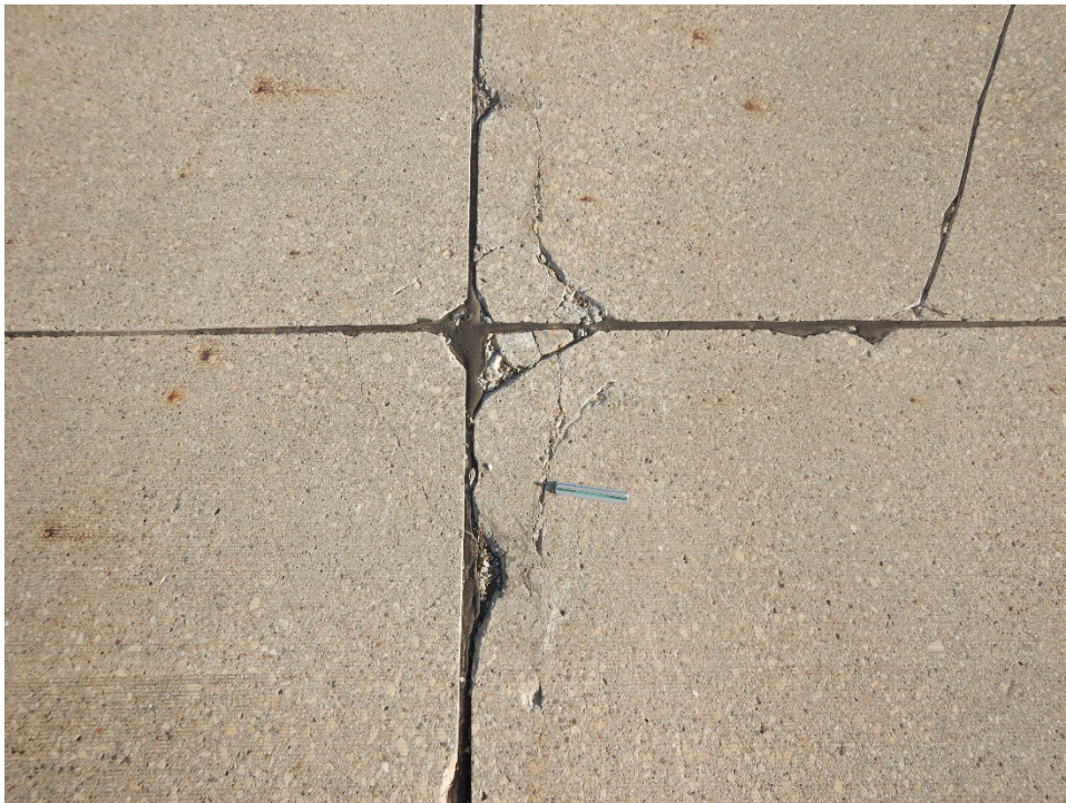
A01OA-01. ASR (Sample Unit No. 05).
