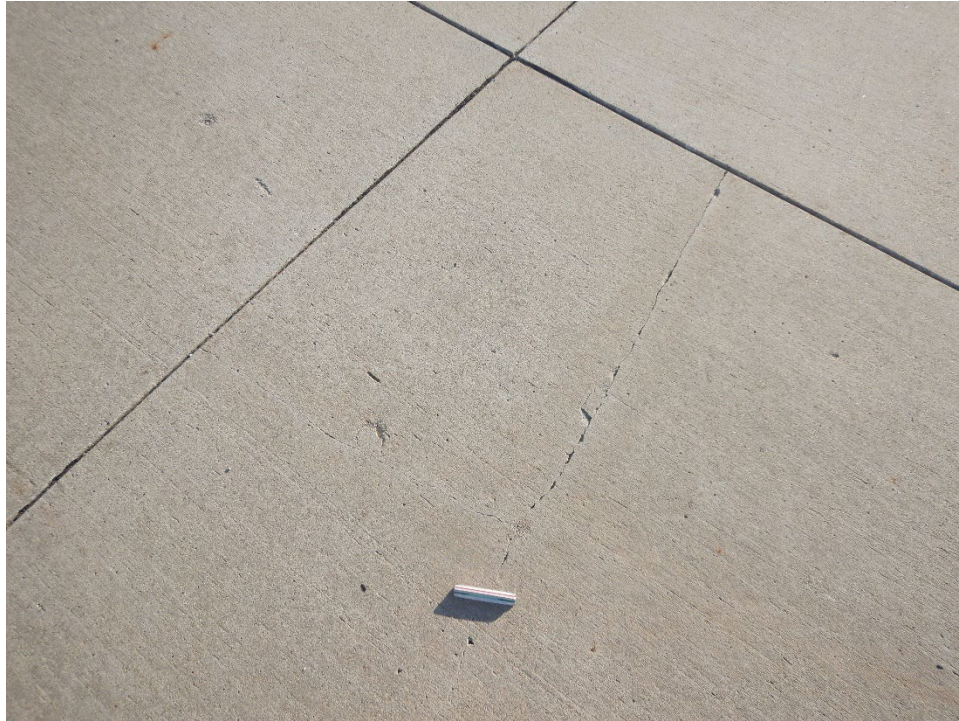
TH01OA-02. Corner Break (Sample Unit No. 02).
