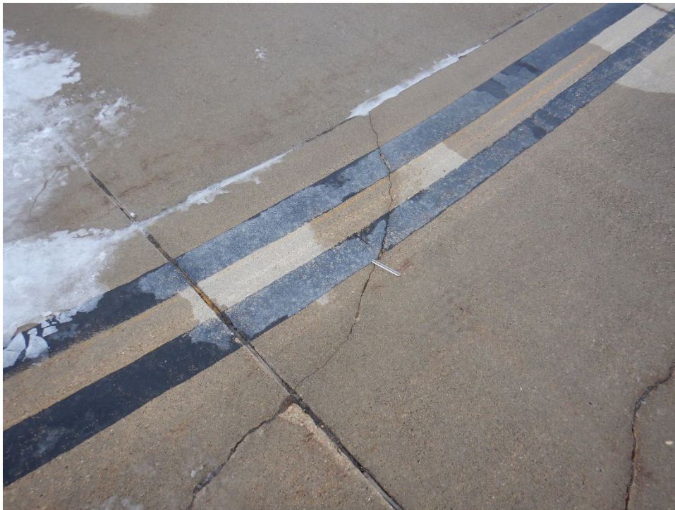
TH01OE-04. Corner Break (Sample Unit No. 03).
