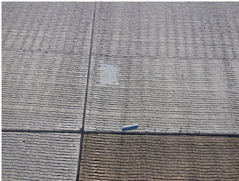
T01OE-01. Small Patching (Sample Unit No. 03).
