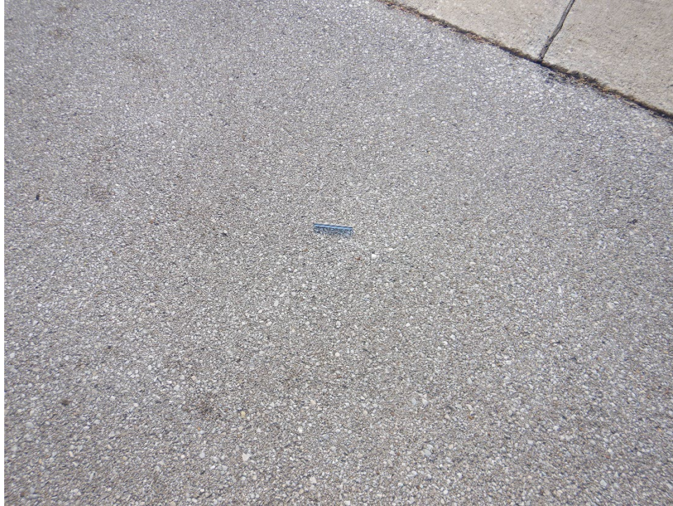
TH01OE-01. Weathering (Sample Unit No. 02).
