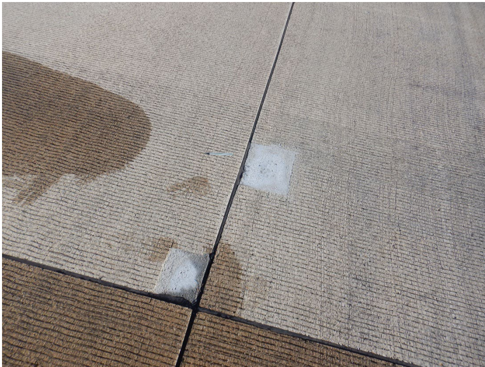
R13OE-01. Small Patching (Sample Unit No. 08).
