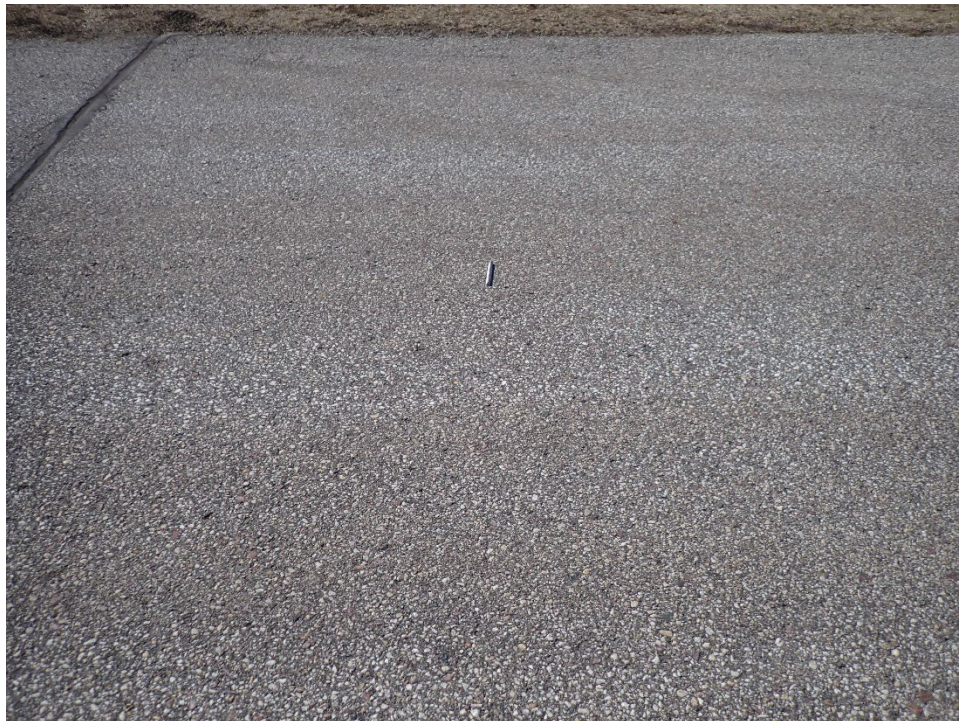
T01MD-01. Raveling (Sample Unit No. 02).
