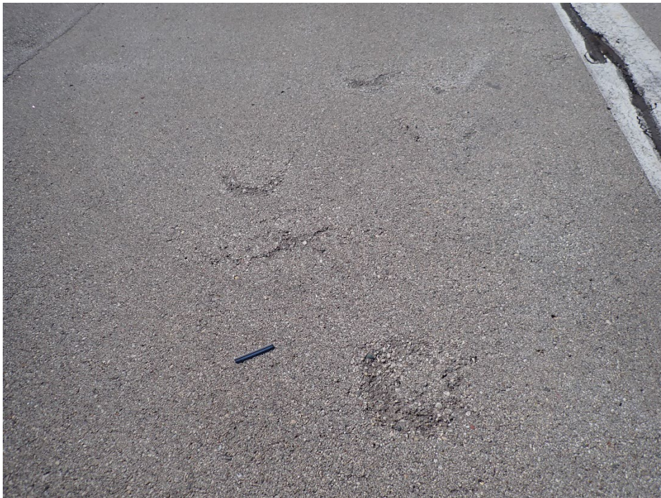
R09MD-02. Raveling (Sample Unit No. 01).
