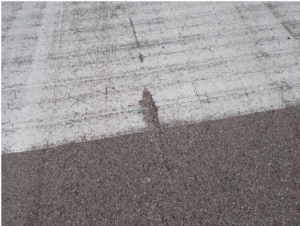
R09MD-03. Raveling (Sample Unit No. 01).
