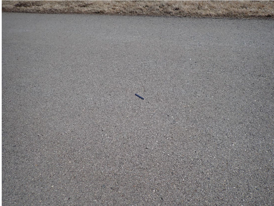
R09MD-01. Weathering (Sample Unit No. 14).
