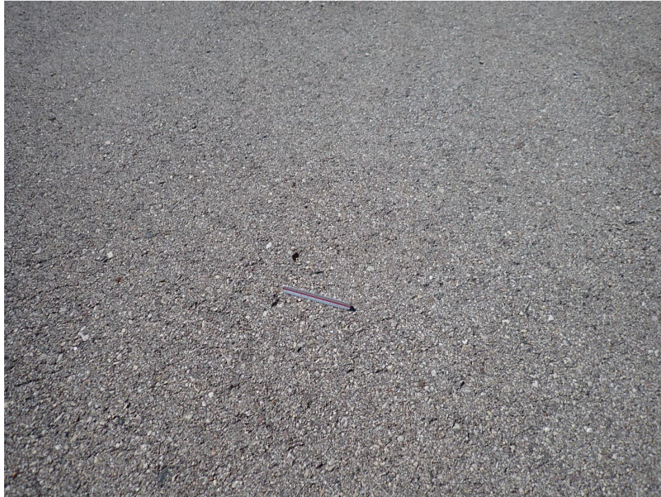
R09MD-03. Weathering (Sample Unit No. 03).
