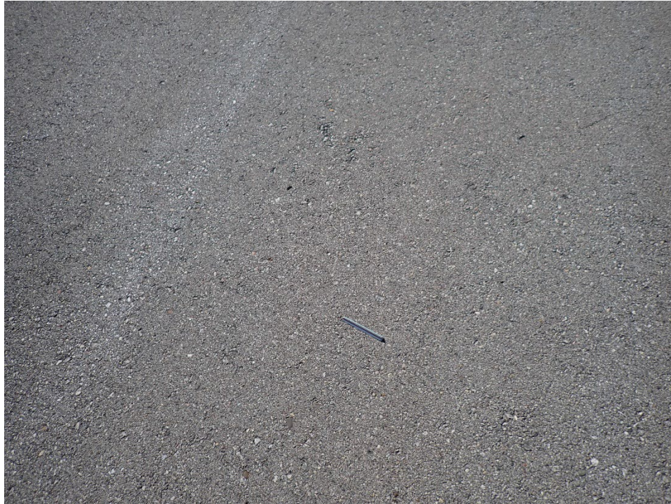
R09MD-02. Weathering (Sample Unit No. 01).
