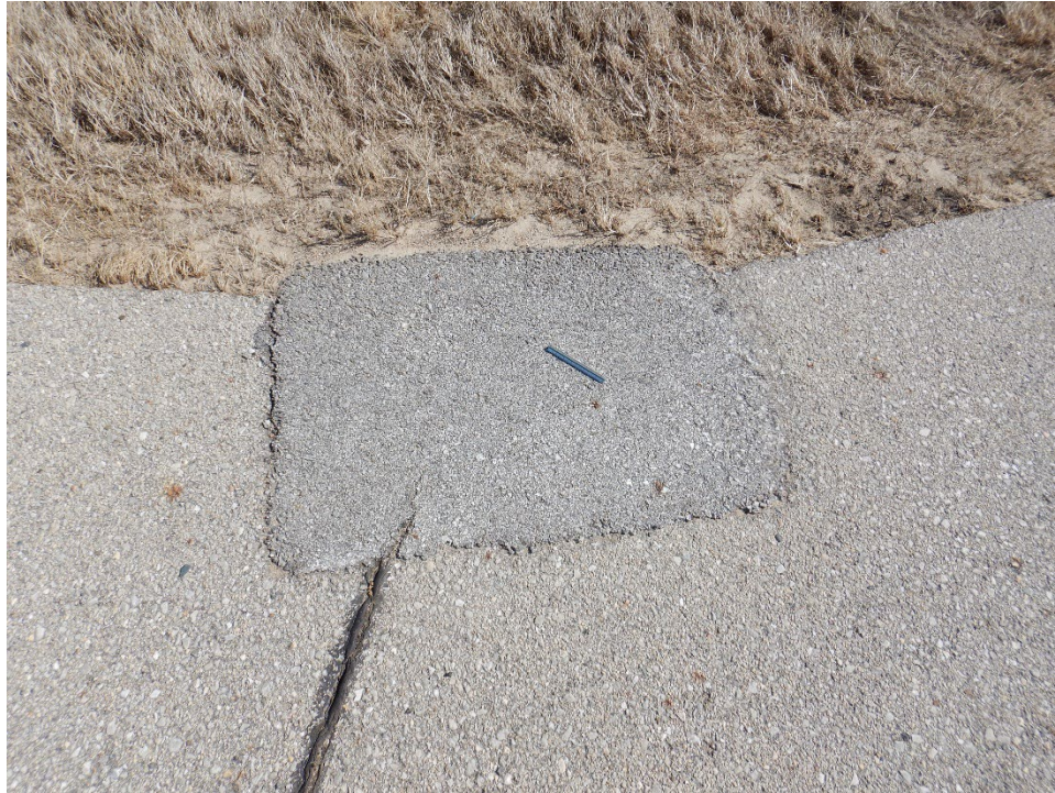
TAMC-10. Patching (Sample Unit No. 10).
