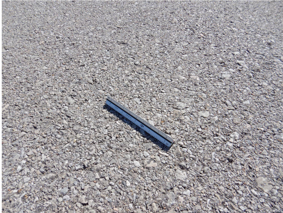
TAMC-30. Weathering (Sample Unit No. 18).
