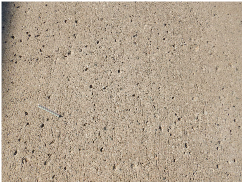
TH01MC-30. Popouts (Sample Unit No. 18).
