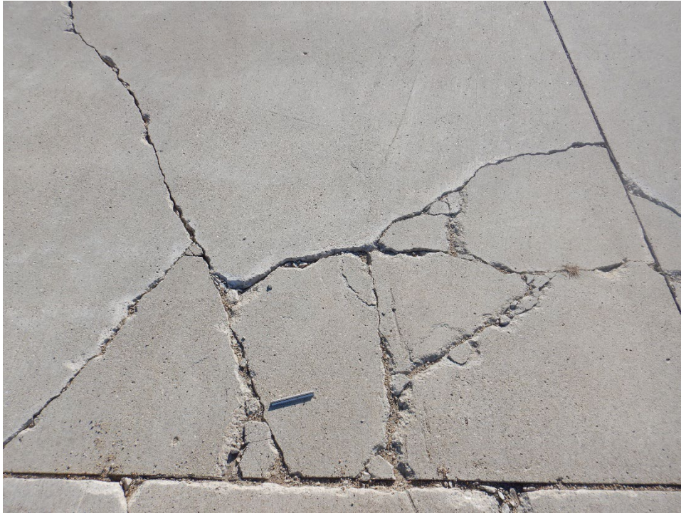
A01MC-70. Shattered Slab (Sample Unit No. 02).
