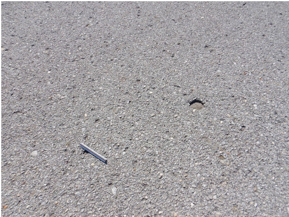
TAMC-20. Raveling (Sample Unit No. 01).
