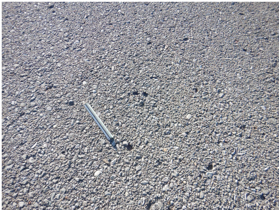
R12MC-20. Raveling (Sample Unit No. 02).
