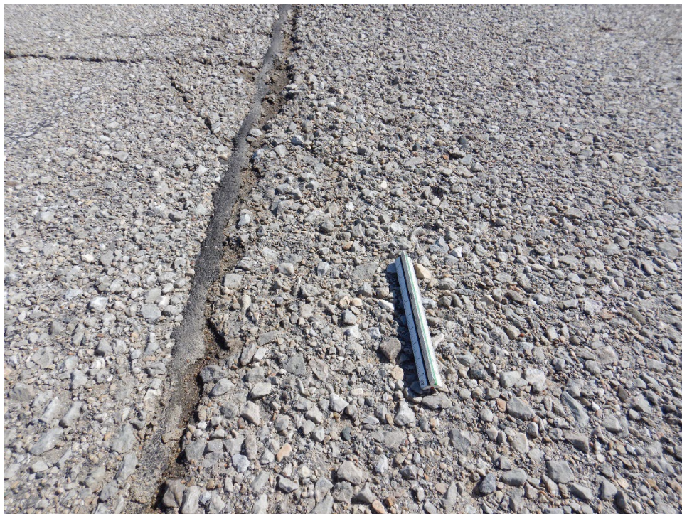
TAMC-10. Weathering (Sample Unit No. 10).
