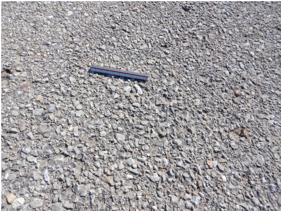
A01MC-50. Weathering (Sample Unit No. 01).
