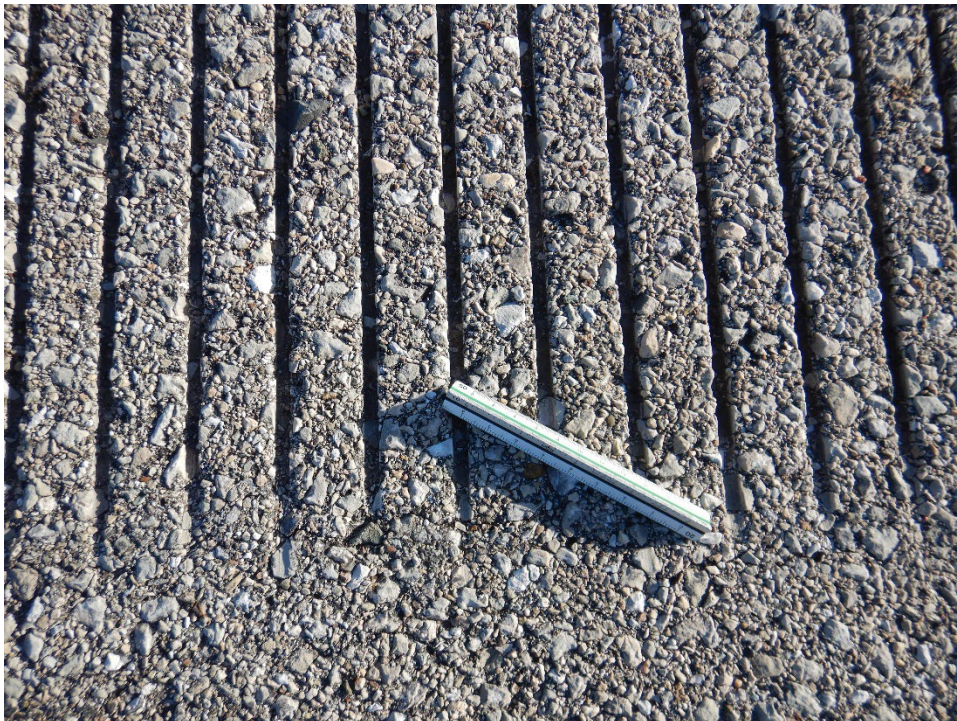
R12MC-10. Weathering (Sample Unit No. 03).
