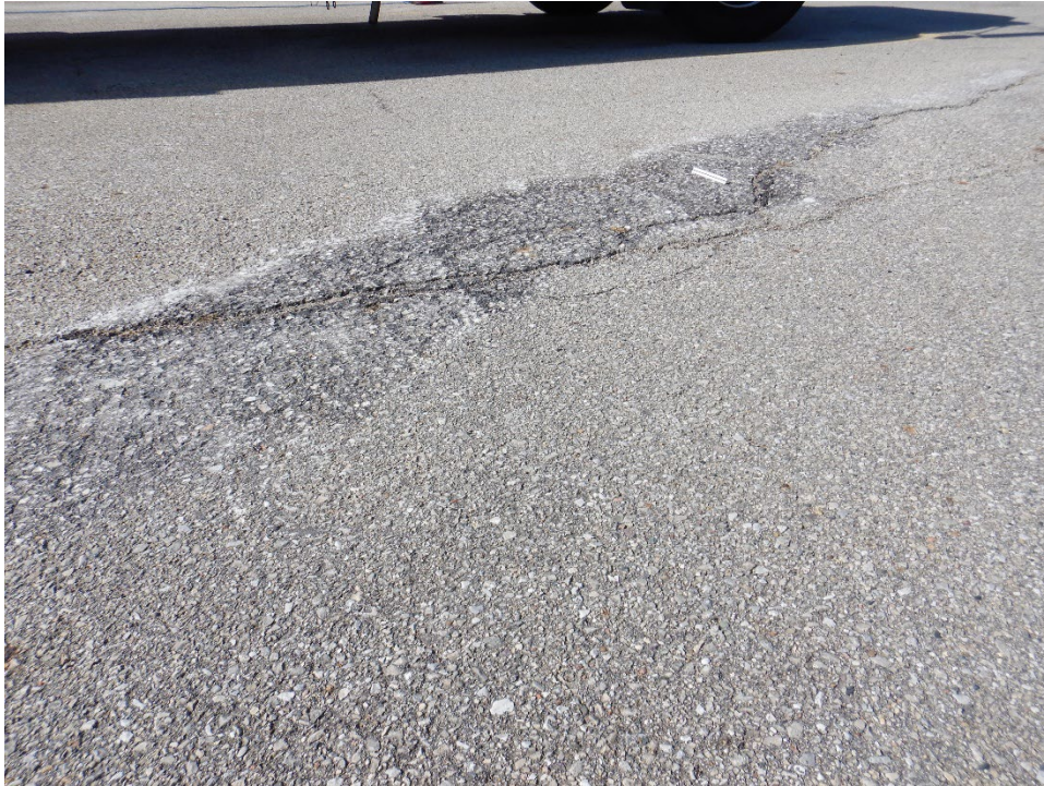
A01MC-60. Swelling (Sample Unit No. 04).
