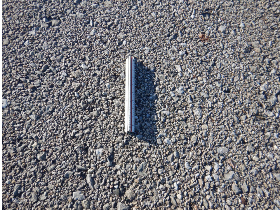
R12MC-20. Weathering (Sample Unit No. 02).
