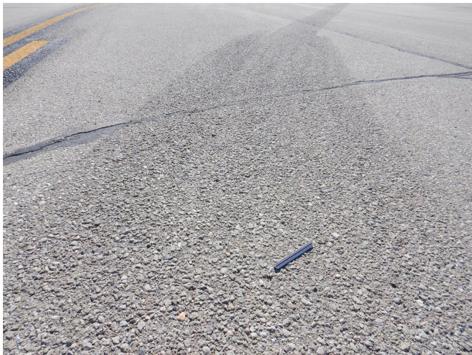
TBMC-10. Weathering (Sample Unit No. 02).
