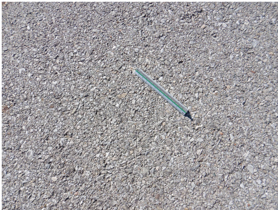
A01MC-35. Weathering (Sample Unit No. 06).
