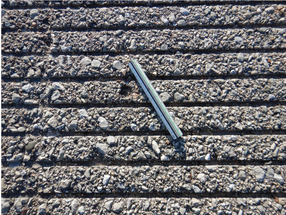
R12MC-10. Raveling (Sample Unit No. 03).
