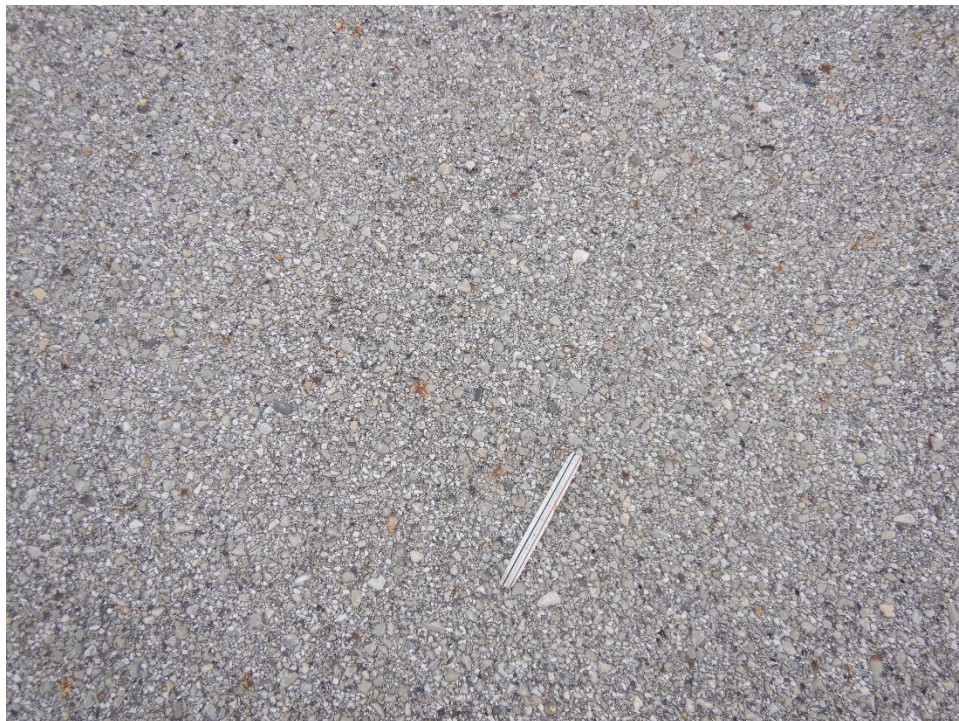
TAMC-20. Weathering (Sample Unit No. 02).
