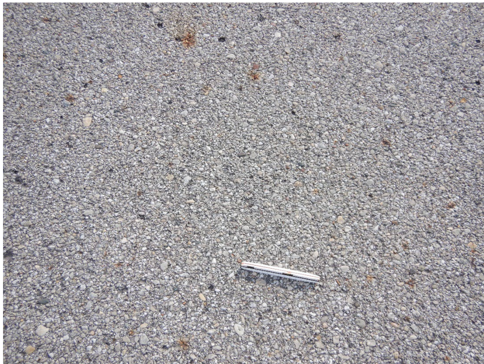
TCMC-20. Weathering (Sample Unit No. 02).
