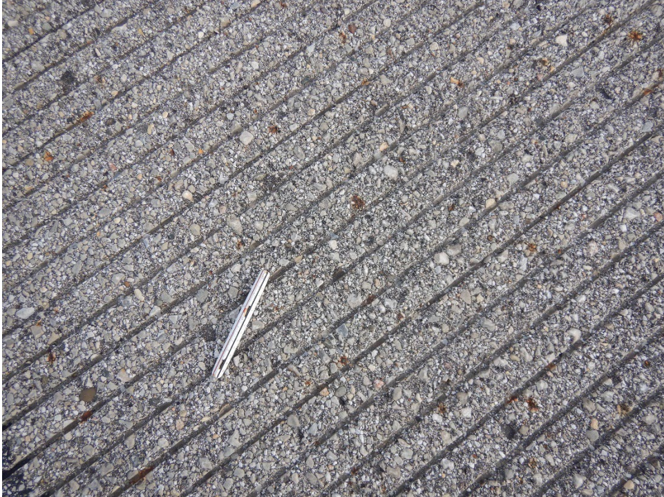
R18MC-20. Weathering (Sample Unit No. 01).
