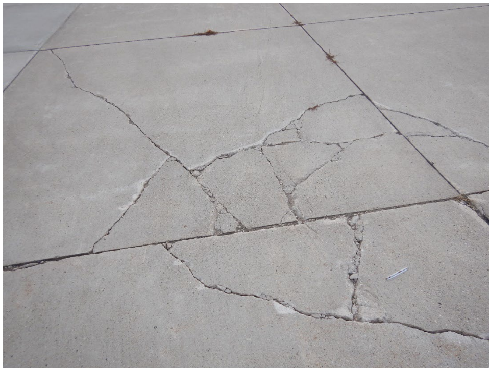
A01MC-70. Shattered Slab (Sample Unit No. 02).
