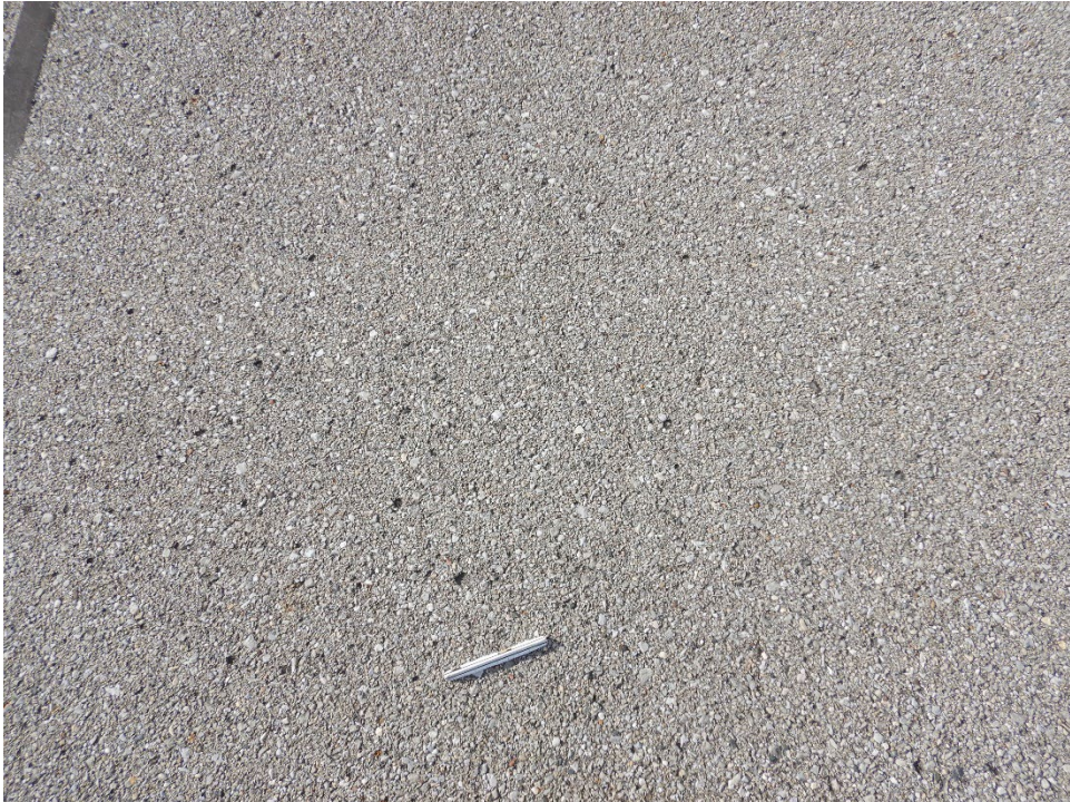
TCMC-10. Weathering (Sample Unit No. 44).
