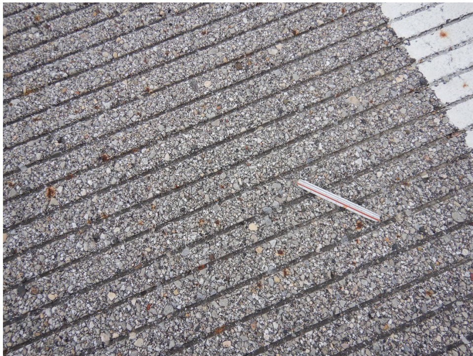
R12MC-40. Weathering (Sample Unit No. 01).
