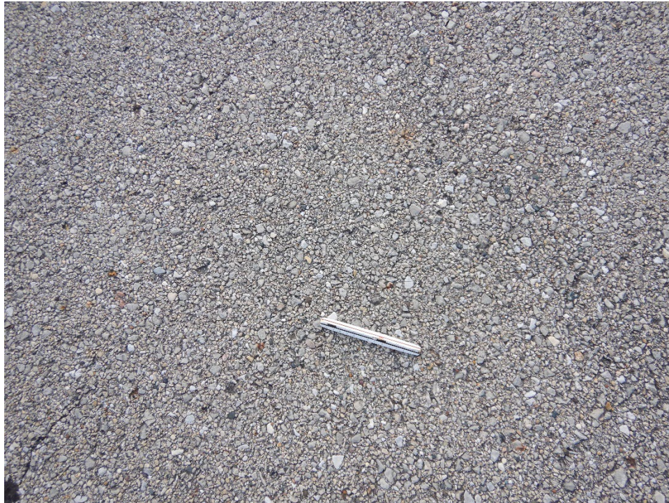
TAMC-10. Weathering (Sample Unit No. 40).
