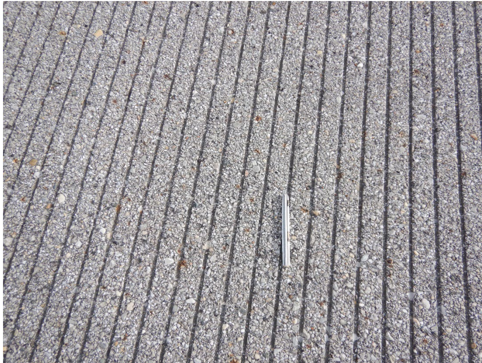
R18MC-30. Weathering (Sample Unit No. 02).
