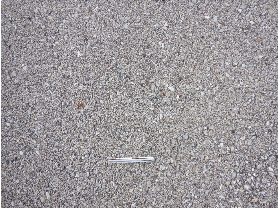
TBMC-30. Weathering (Sample Unit No. 04).
