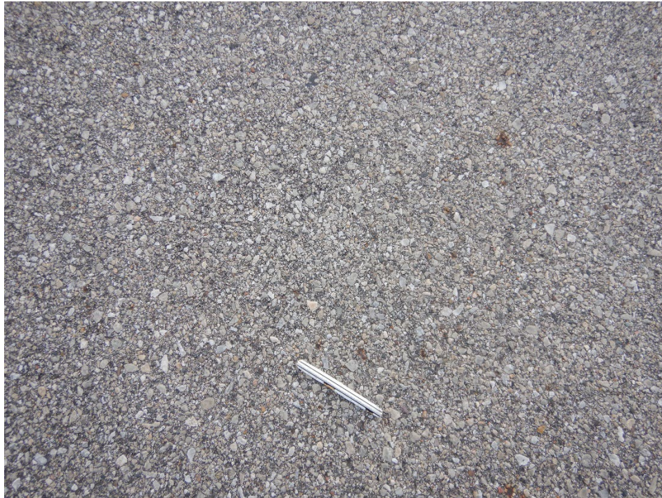
A01MC-60. Weathering (Sample Unit No. 01).
