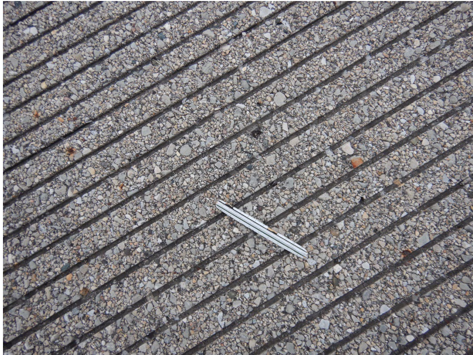
R12MC-10. Weathering (Sample Unit No. 43).
