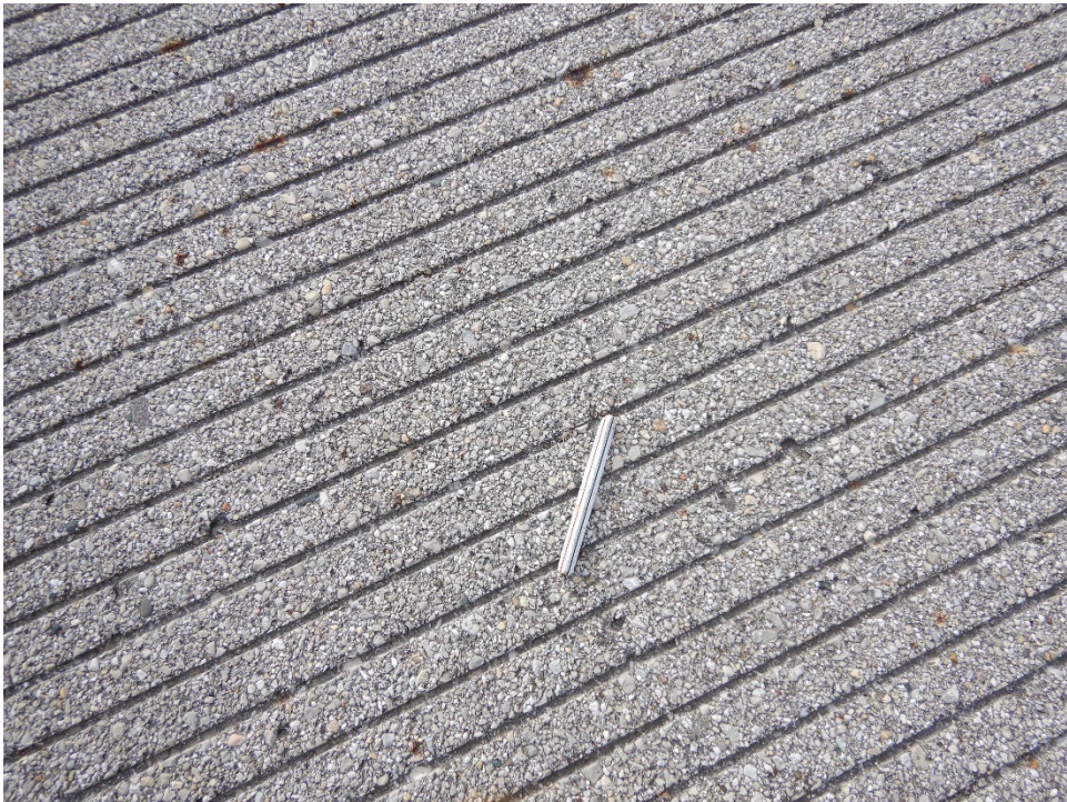
R18MC-40. Weathering (Sample Unit No. 02).
