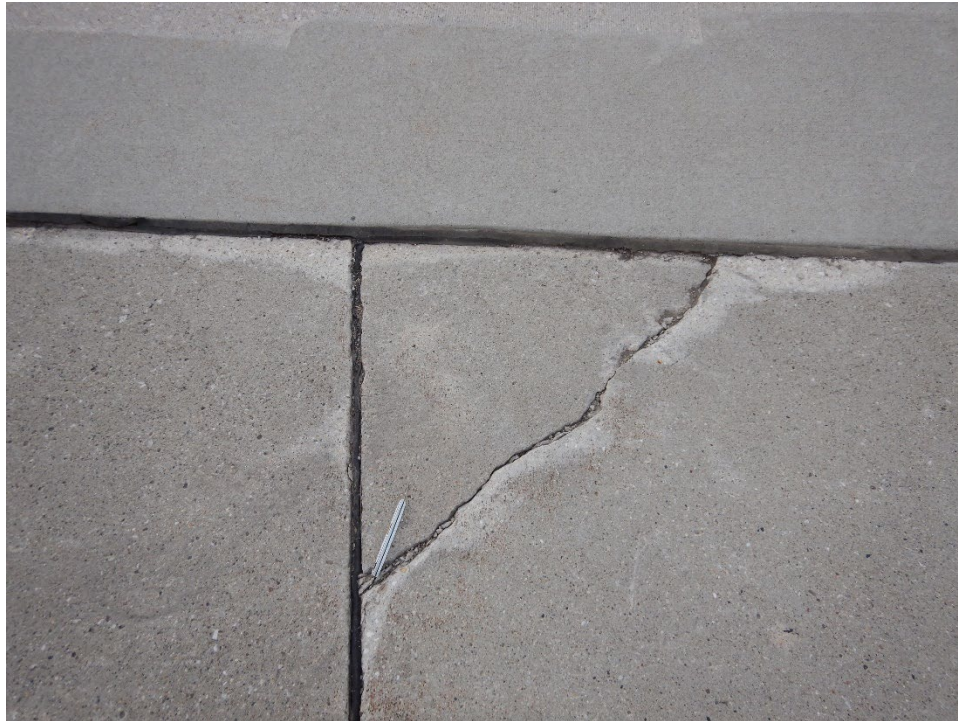
A01MC-70. Corner Break (Sample Unit No. 01).
