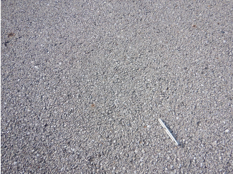
A01MC-50. Weathering (Sample Unit No. 01).
