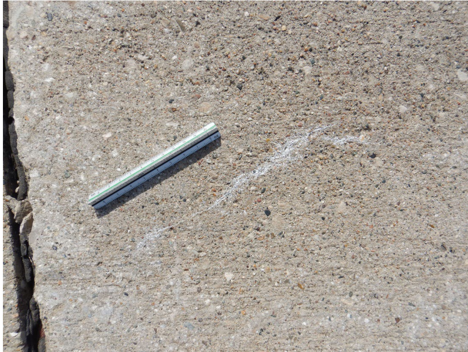
A01MT-01. ASR (Sample Unit No. 11).
