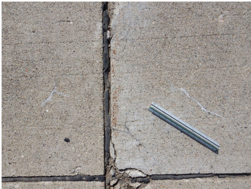
A01MT-01. ASR (Sample Unit No. 04).
