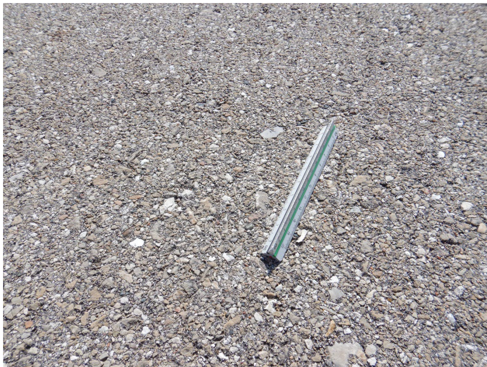
T01MT-01. Weathering (Sample Unit No. 08).
