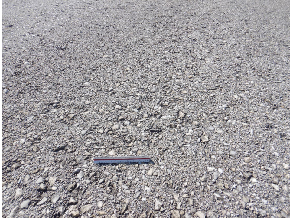
R13MT-03. Raveling (Sample Unit No. 01).
