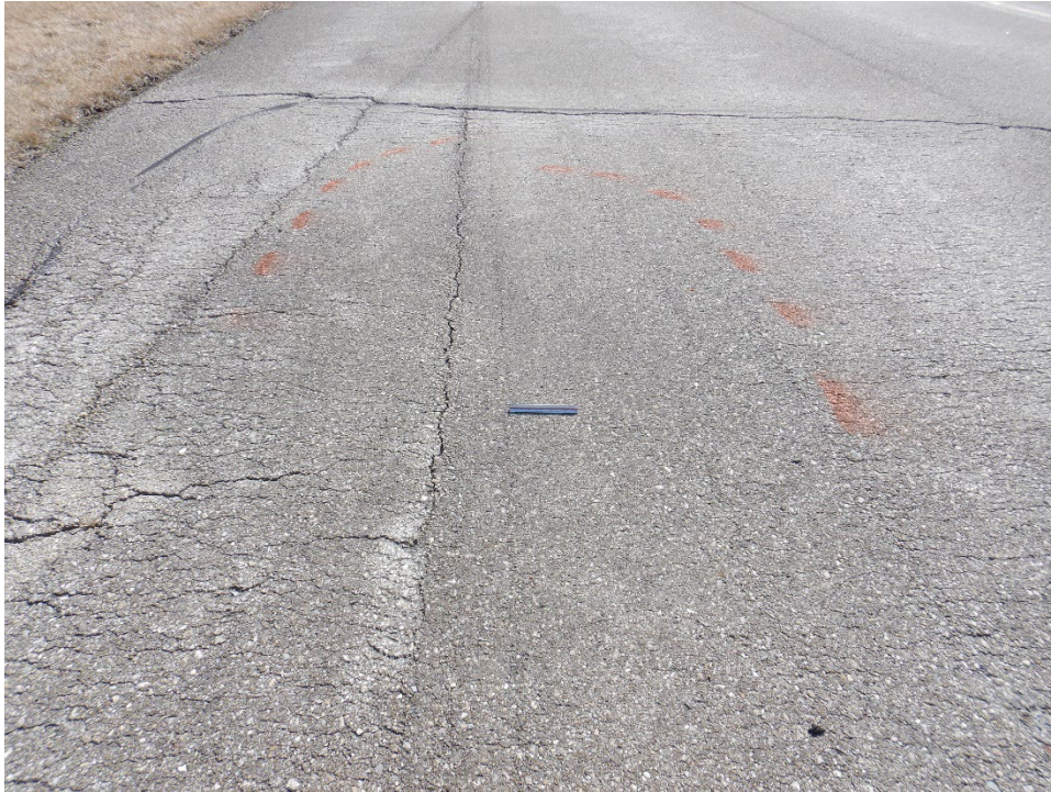
T03MT-03. Depression (Additional Sample Unit No. 05).
