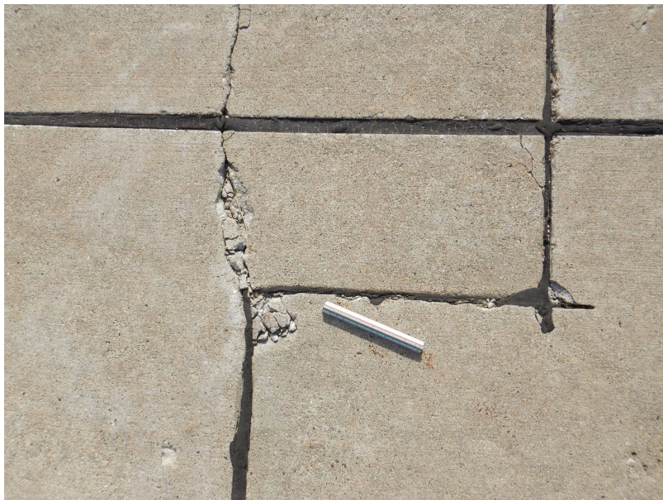
TH01MT-01. Small Patching (Sample Unit No. 11).
