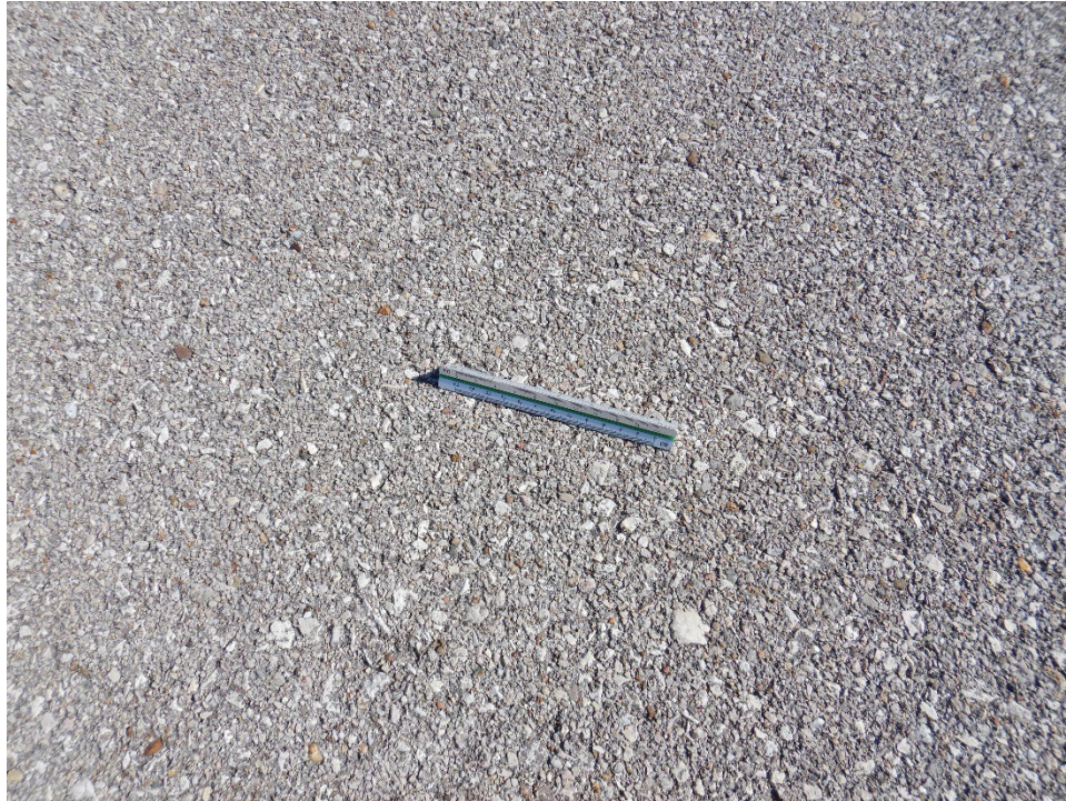
R17MR-03. Weathering (Sample Unit No. 03).
