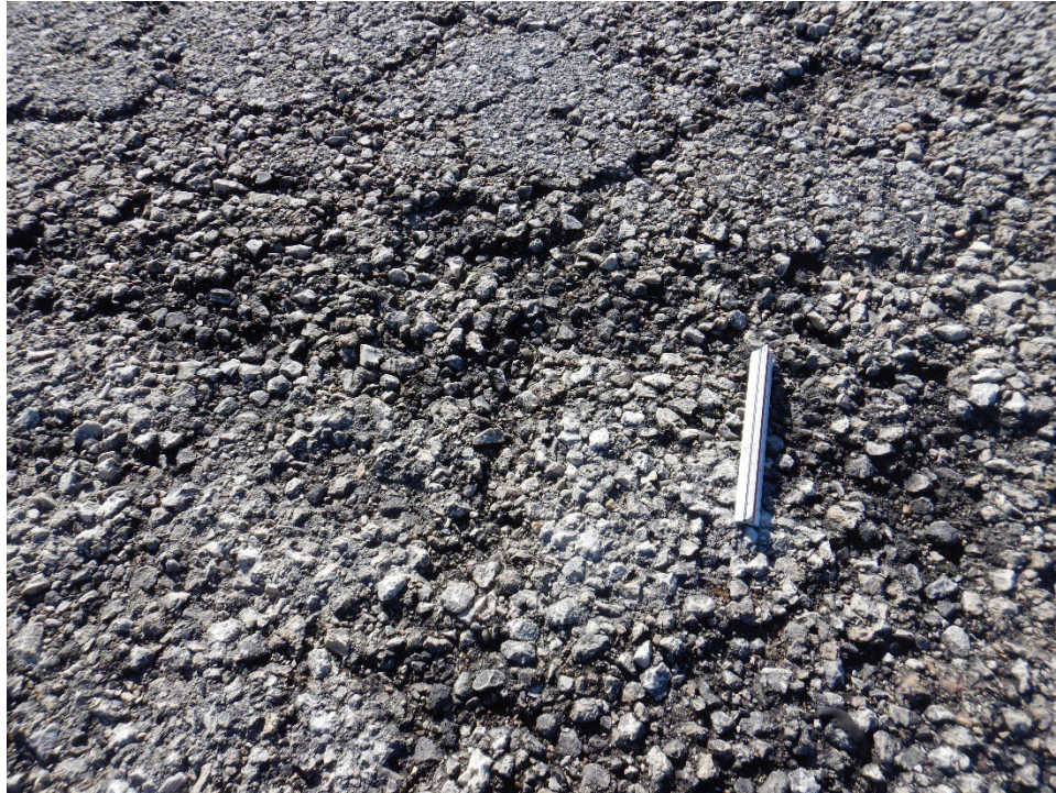
A01MR-01. Raveling (Sample Unit No. 04).
