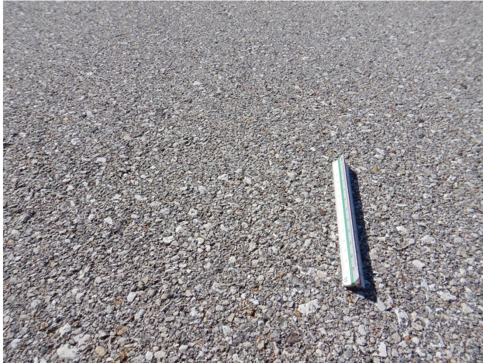
R17MR-02. Weathering (Sample Unit No. 35).
