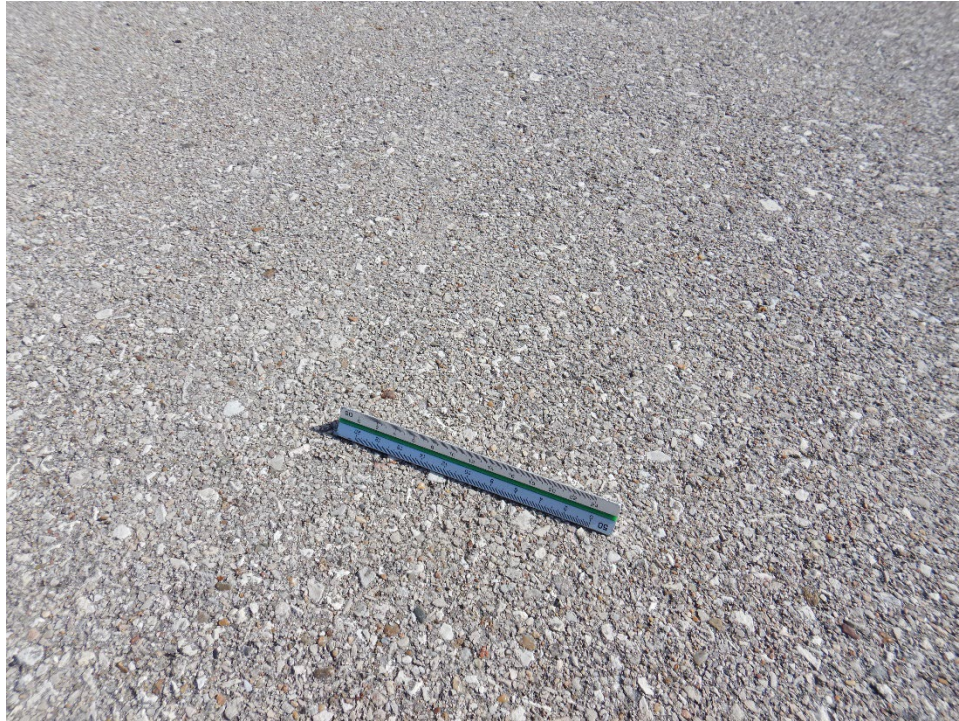
R17MR-04. Weathering (Sample Unit No. 04).
