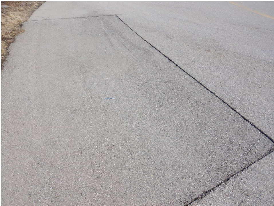
R17MR-04. Patching (Sample Unit No. 01).
