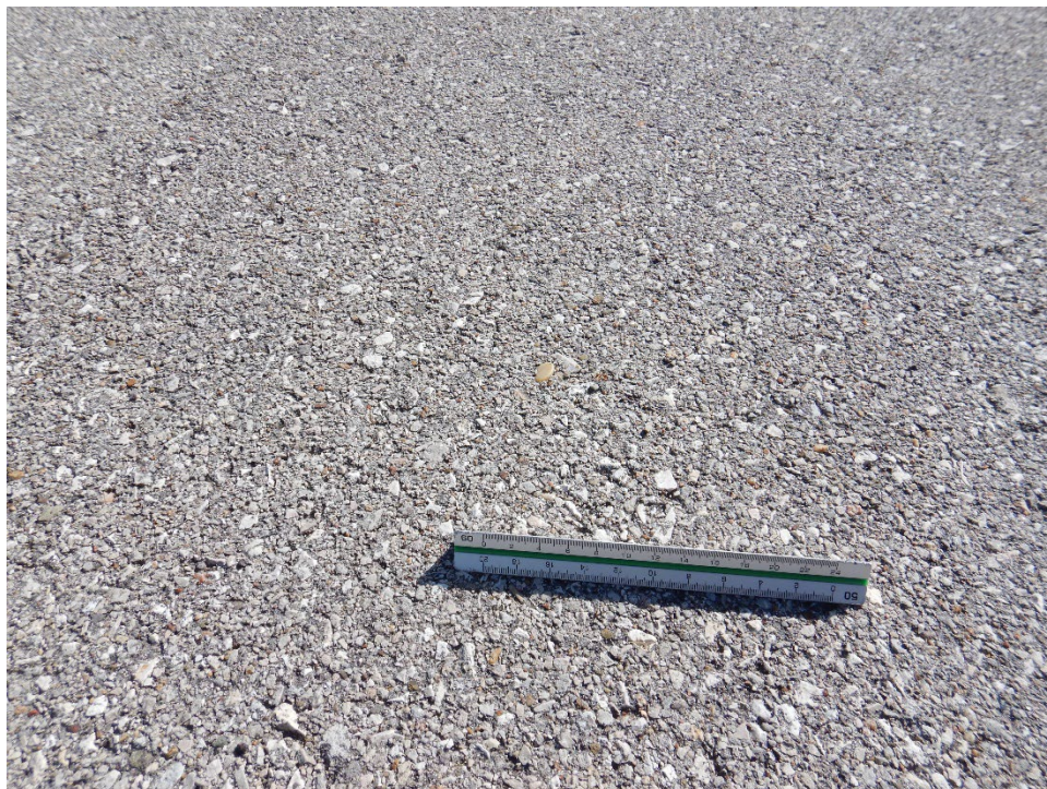
R17MR-01. Weathering (Sample Unit No. 15).
