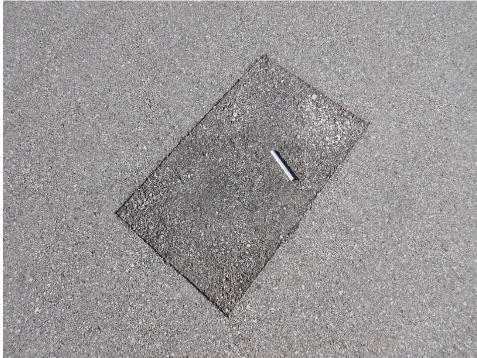
R17MR-01. Patching (Sample Unit No. 08).
