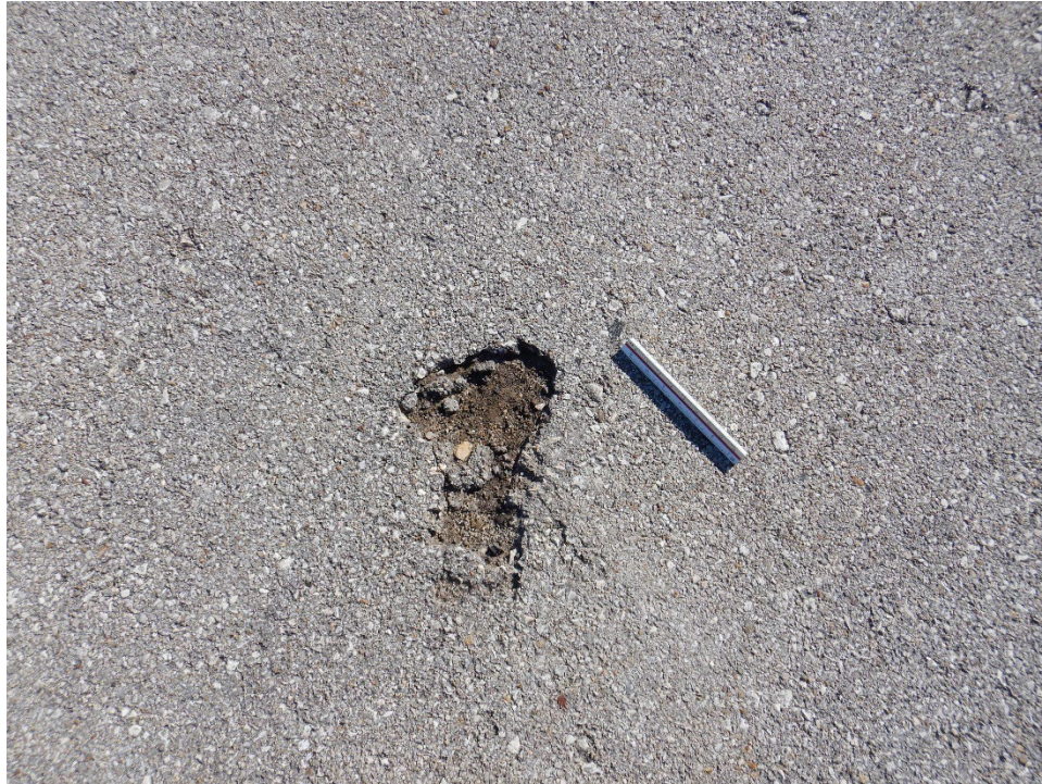
R17MR-03. Raveling (Sample Unit No. 06).
