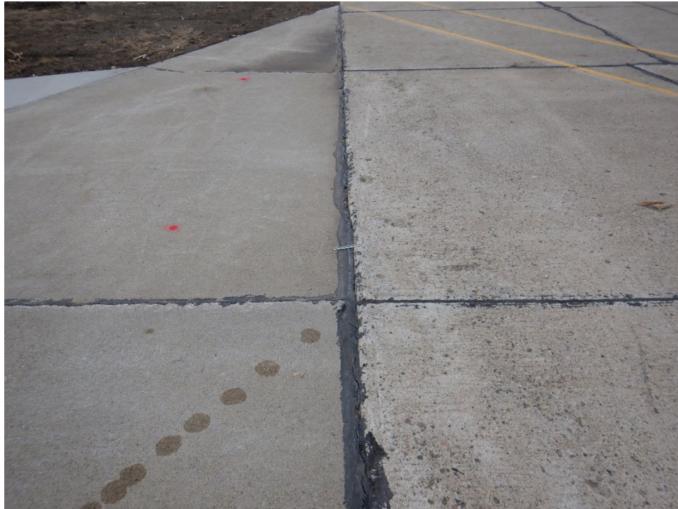
TH01LE-01. Faulting (Sample Unit No. 01).
