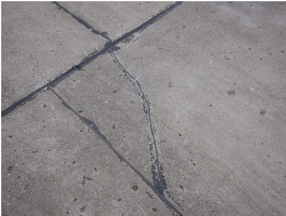
TH01LE-02. Corner Break (Sample Unit No. 01).
