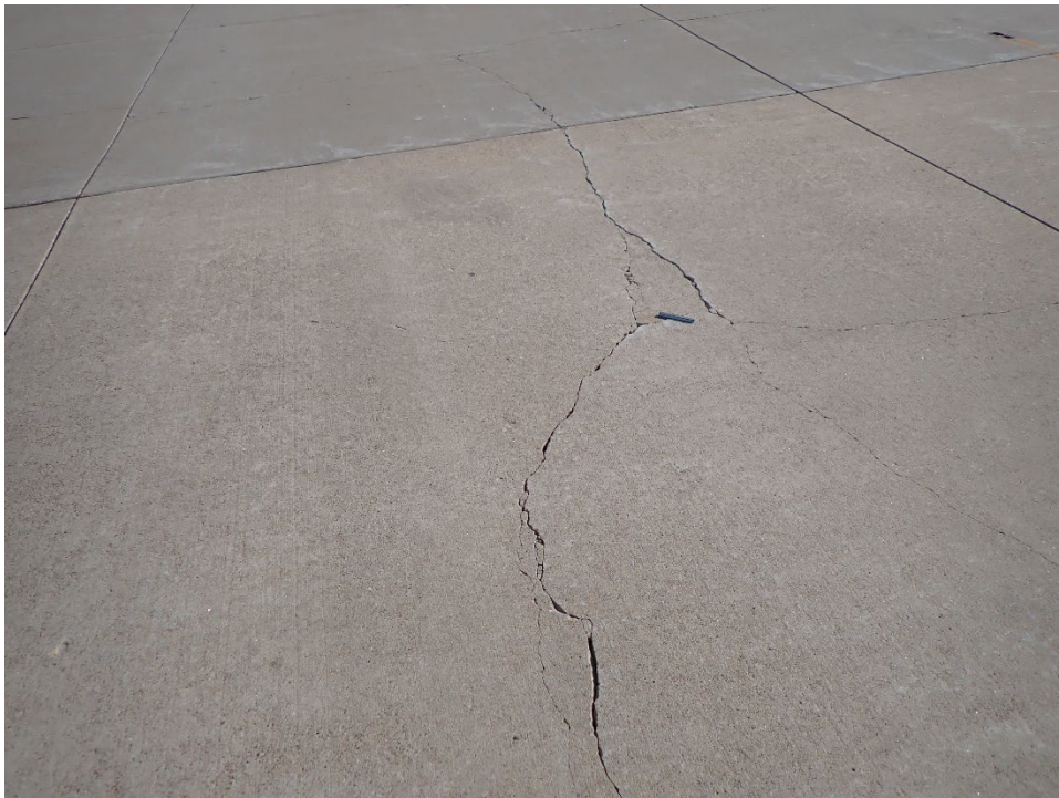
A02KN-02. Shattered Slab (Sample Unit No. 03).
