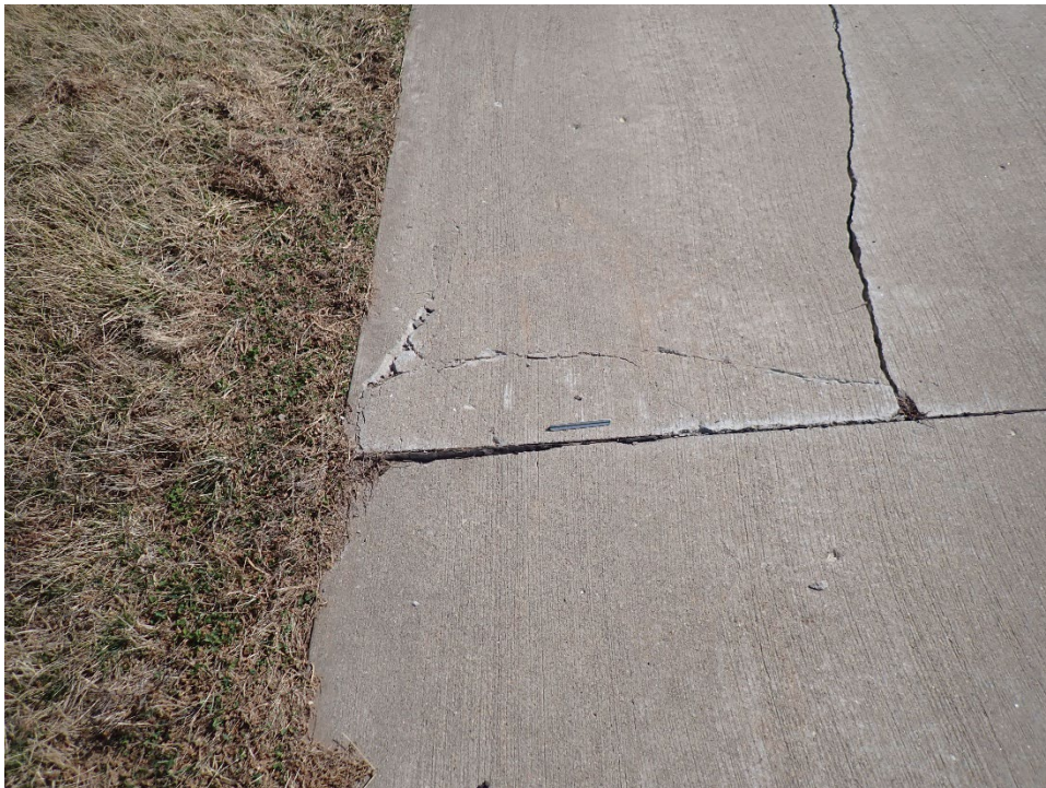
TBKN-01. Blow-Up (Sample Unit No. 12).
