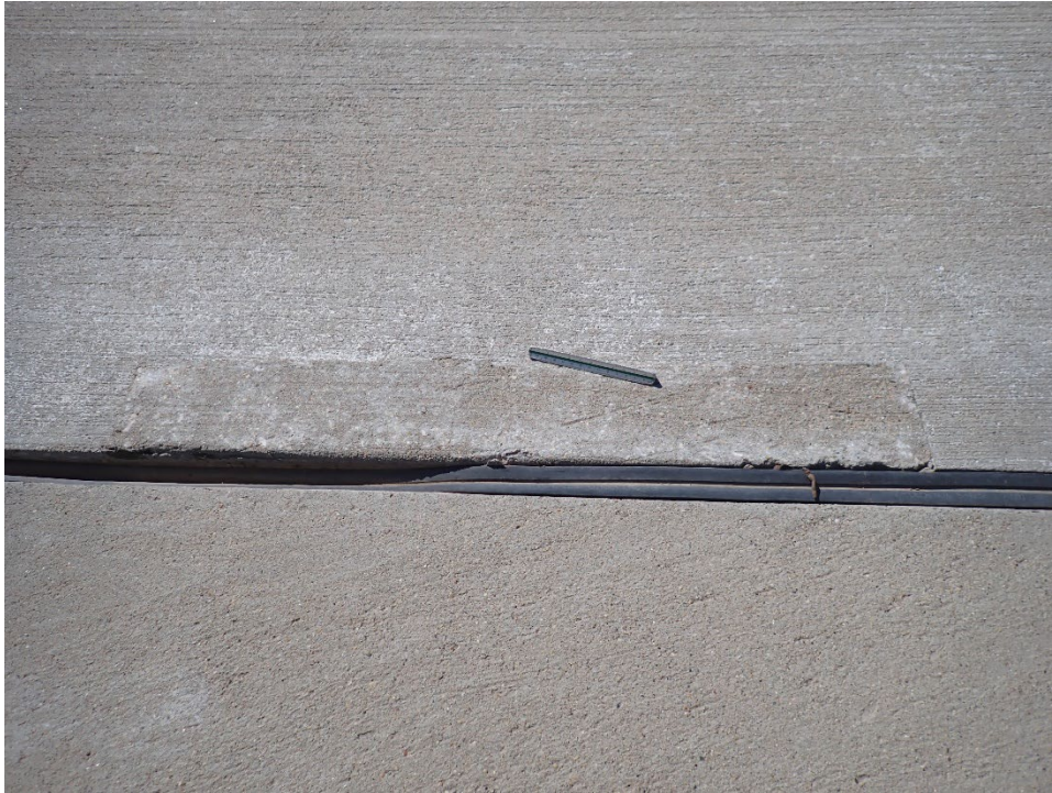
R15KN-01. Small Patching (Sample Unit No. 14).
