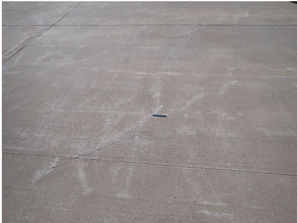
A01KN-01. Shattered Slab (Sample Unit No. 13).
