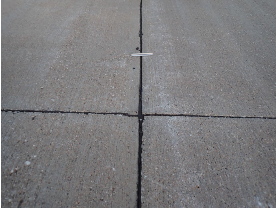
R14JE-02. Faulting (Sample Unit No. 04).
