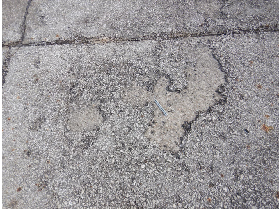
TH01IC-02. Raveling (Sample Unit No. 02).
