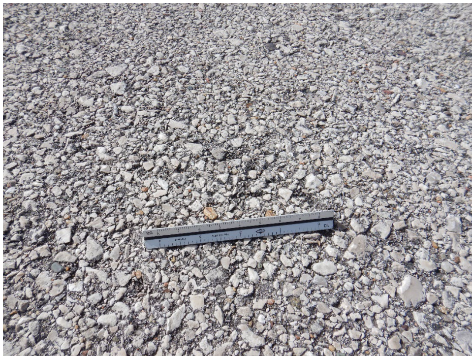
TBIC-04. Weathering (Sample Unit No. 01).
