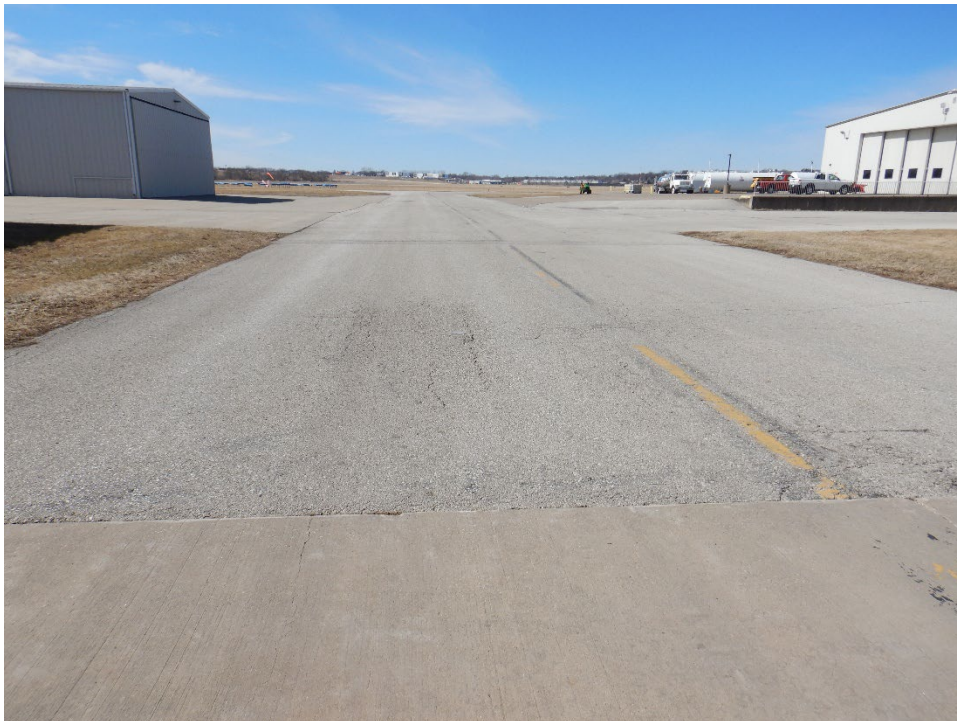
TH02IC-01. Rutting (Sample Unit No. 03).
