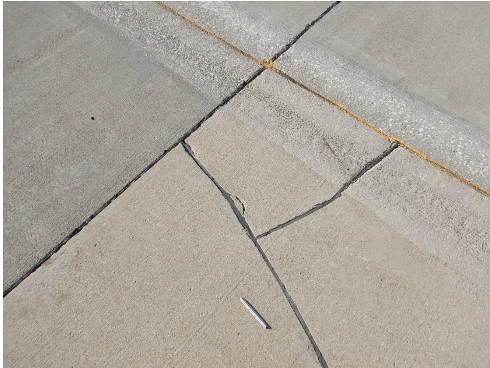
TH01IN-02. Corner Break (Sample Unit No. 03).
