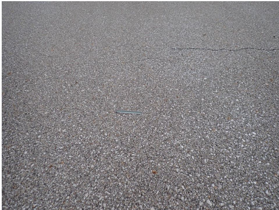
R12IG-03. Weathering (Sample Unit No. 01).
