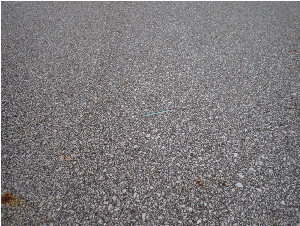
R12IG-02. Weathering (Sample Unit No. 22).
