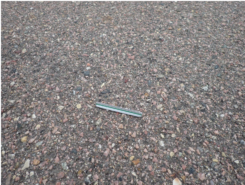
R12IG-01. Weathering (Sample Unit No. 04).
