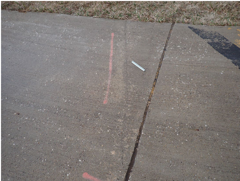
T02HL-03. Corner Break (Sample Unit No. 05).
