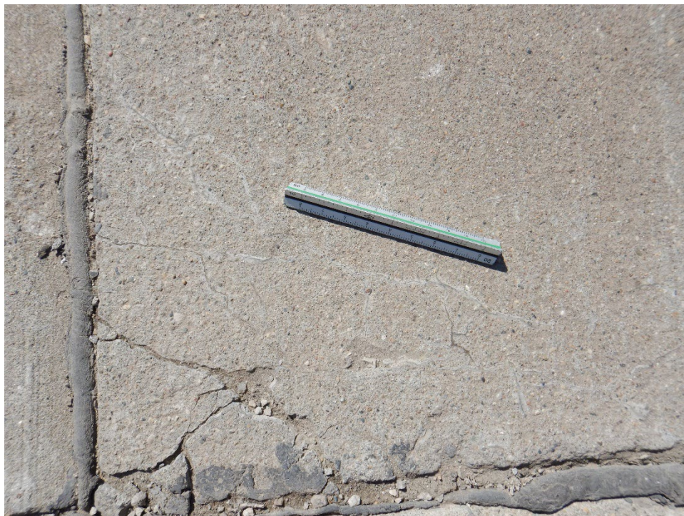
A01GL-02. ASR (Sample Unit No. 01).
