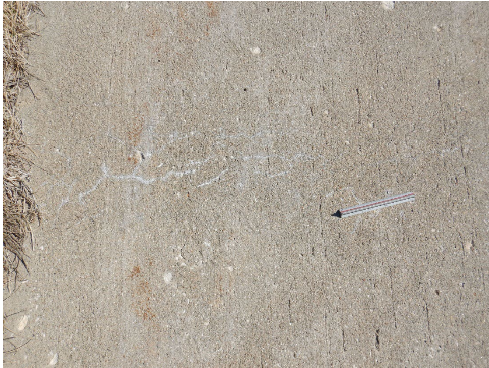
T02GL-01. ASR (Sample Unit No. 04).
