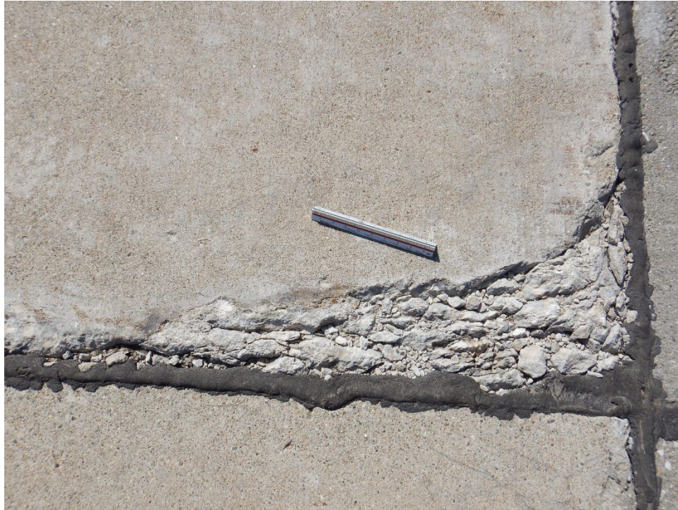
A01GL-01. ASR (Sample Unit No. 06).
