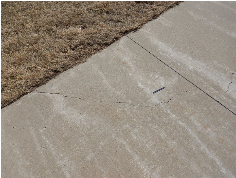
TH01GL-01. Corner Break (Sample Unit No. 08).
