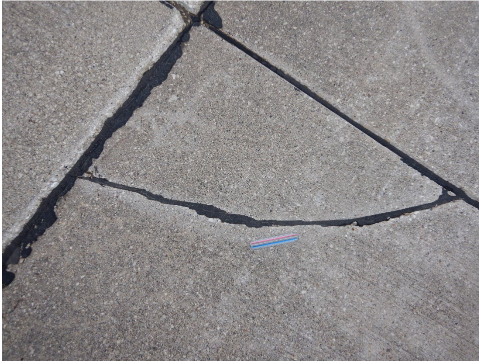
T01GR-01. Corner Break (Sample Unit No. 02).
