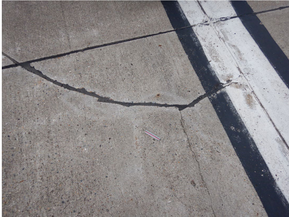
R14GR-03. Corner Break (Sample Unit No. 01).
