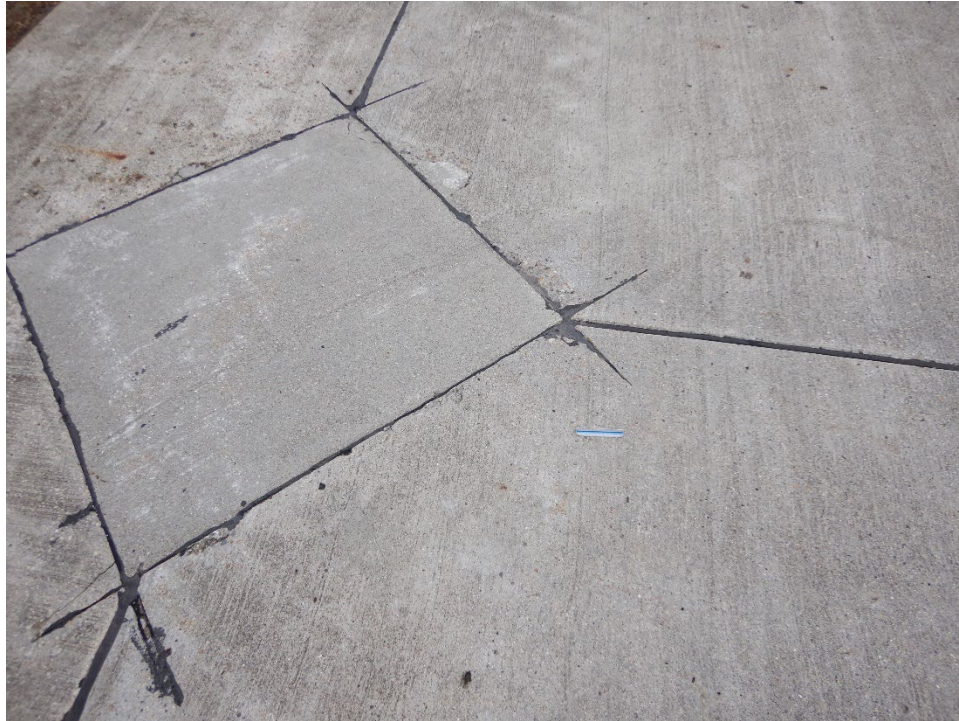
R14GR-02. Small Patching (Sample Unit No. 02).
