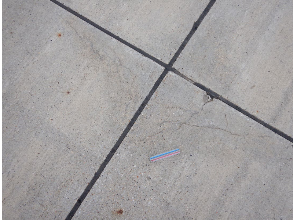
T03GR-01. ASR (Sample Unit No. 02).
