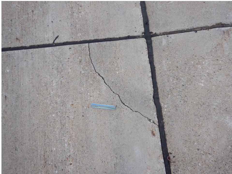
T03GR-01. Corner Break (Sample Unit No. 05).
