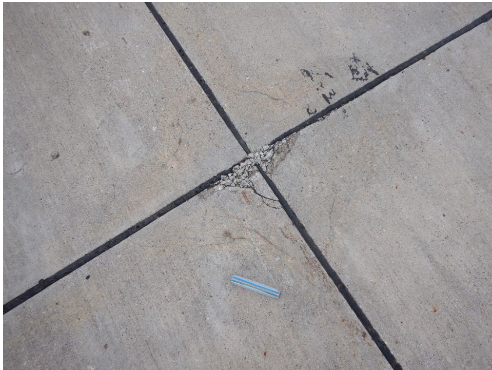
T02GR-01. ASR (Sample Unit No. 15).
