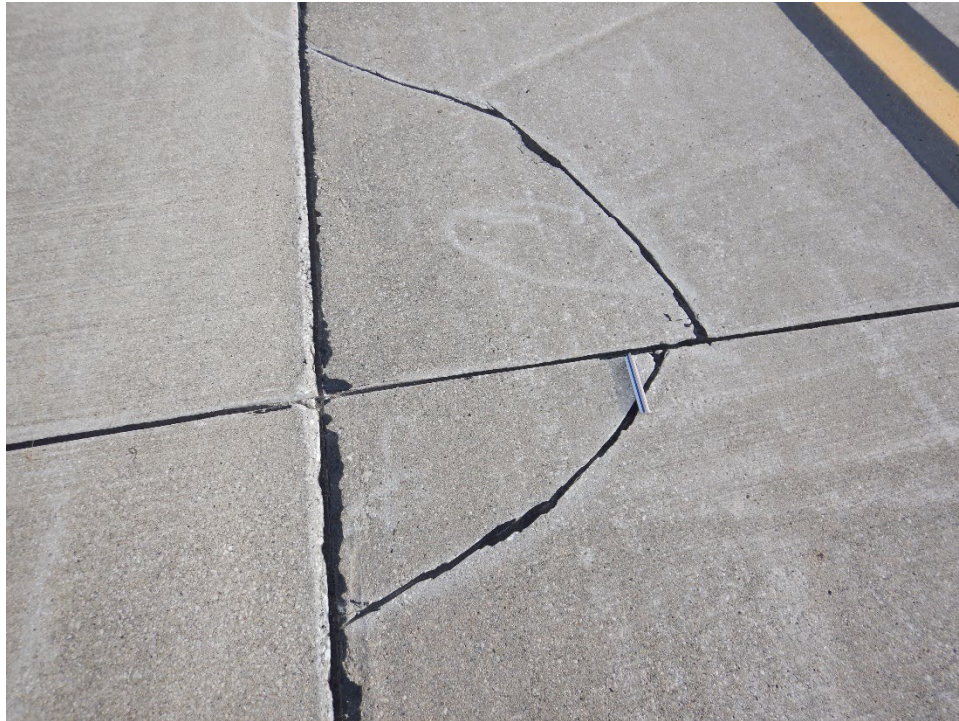
T01GR-01. Corner Break (Sample Unit No. 02).
