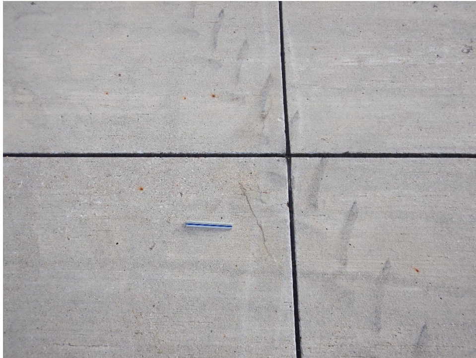
T03GR-01. ASR (Sample Unit No. 02).
