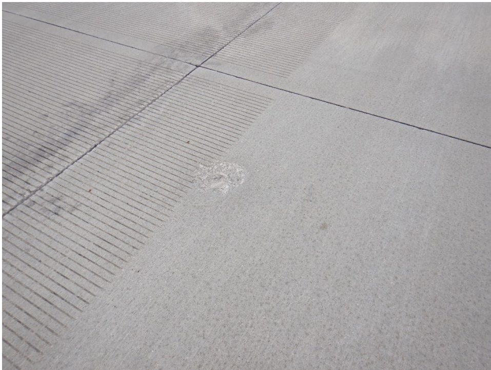
R12FD-04. Scaling (Sample Unit No. 18).
