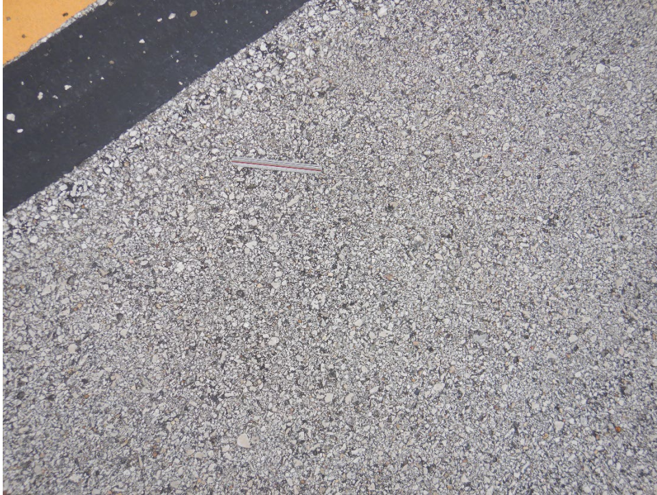
TDFD-02. Weathering (Sample Unit No. 02).
