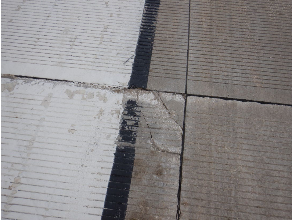
R12FD-03. Small Patching (Sample Unit No. 04).
