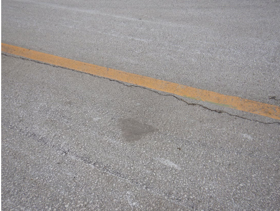
TH01FD-01. Depression (Sample Unit No. 07).
