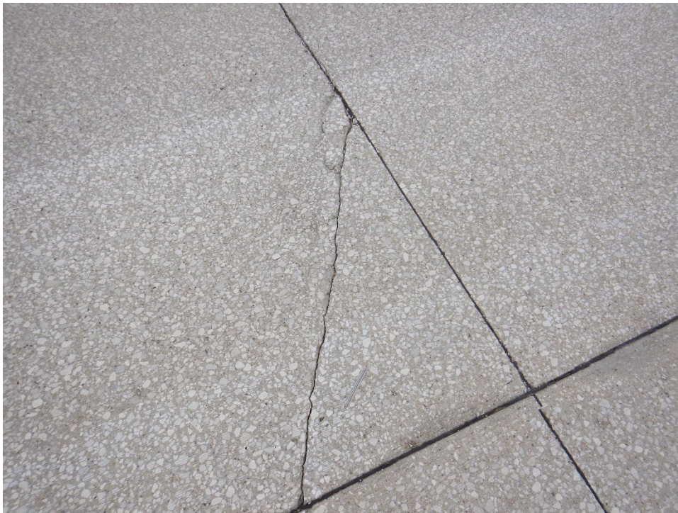
TAFD-01. Corner Break (Sample Unit No. 10).
