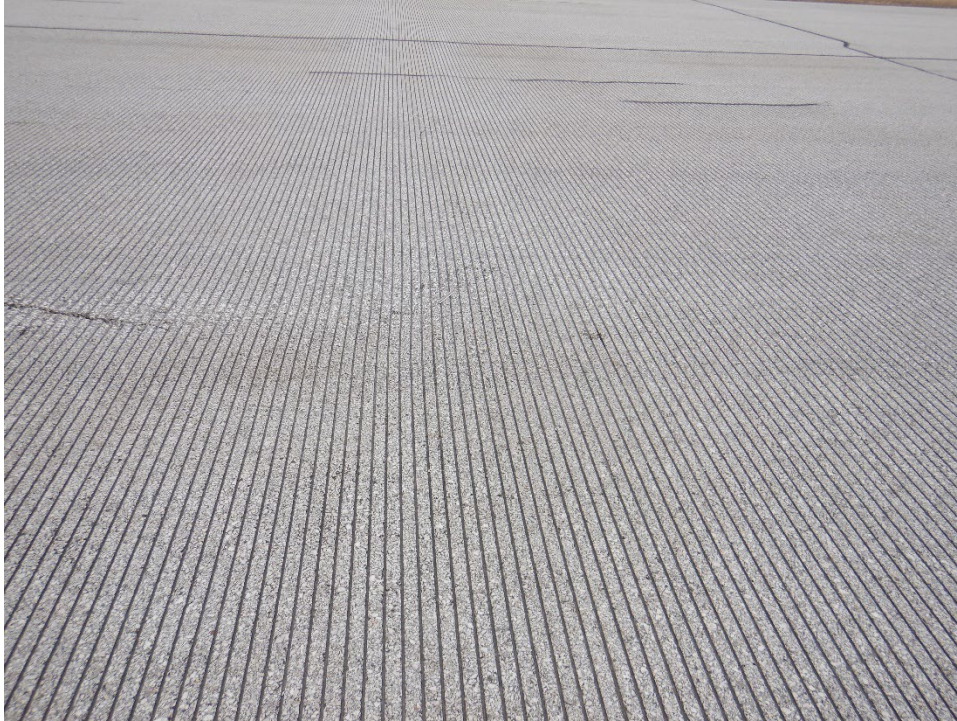
R12FD-02. Swelling (Additional Sample Unit No. 26).
