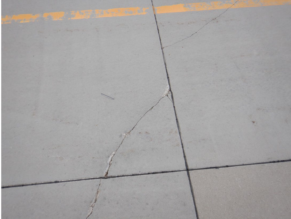
TH01FD-03. Corner Break (Sample Unit No. 06).
