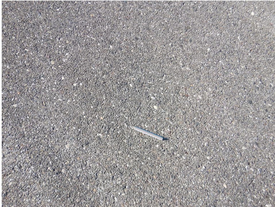
R09FC-01. Weathering (Sample Unit No. 11).
