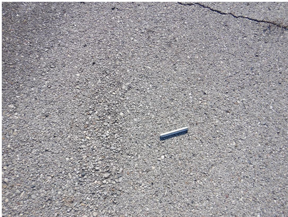
R15FC-03. Weathering (Sample Unit No. 01).
