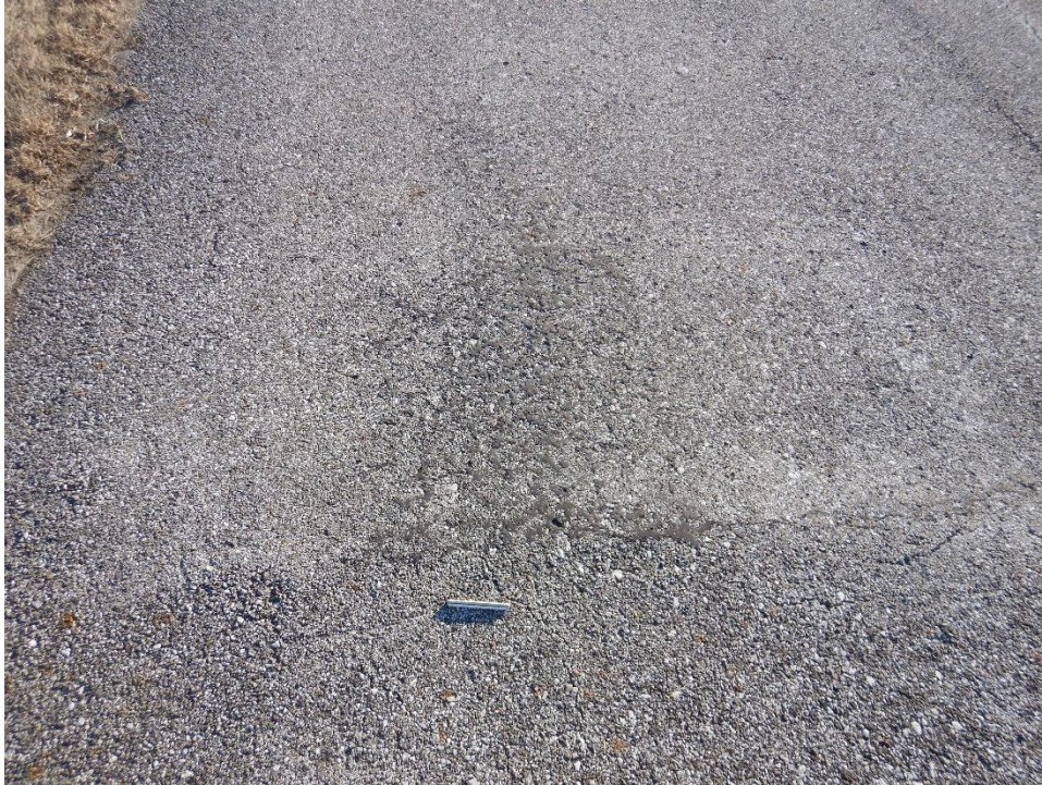
T02FC-01. Bleeding (Sample Unit No. 04).
