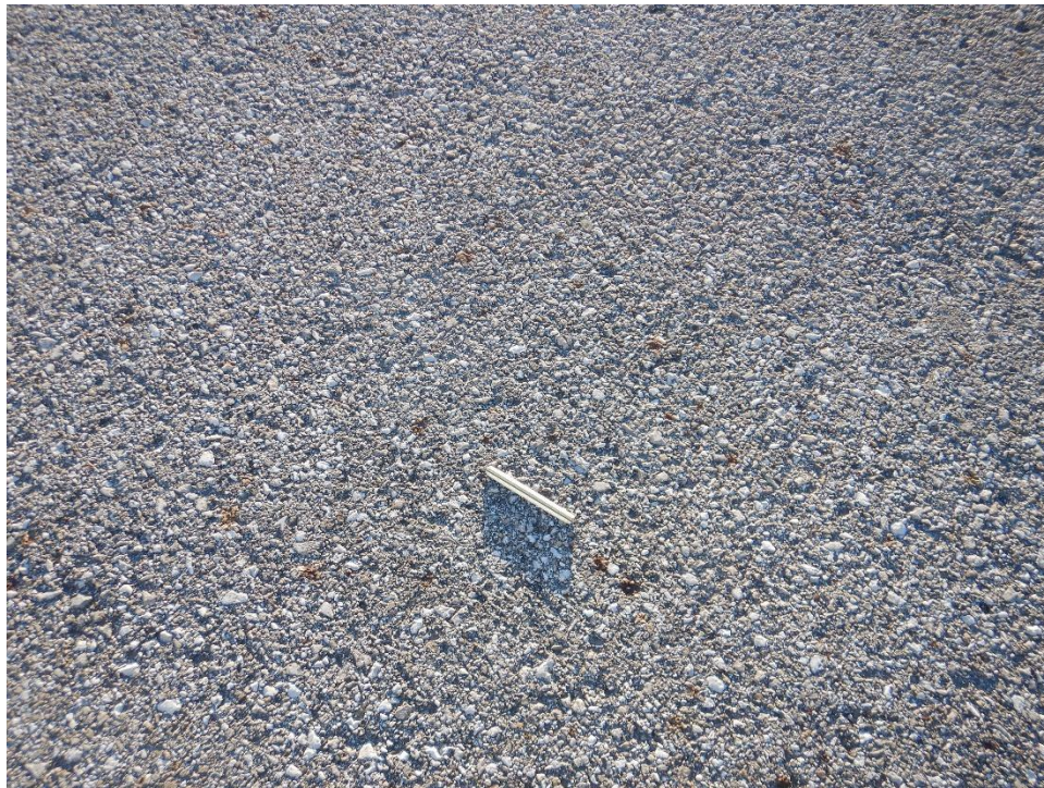
TH01FC-03. Weathering (Sample Unit No. 01).
