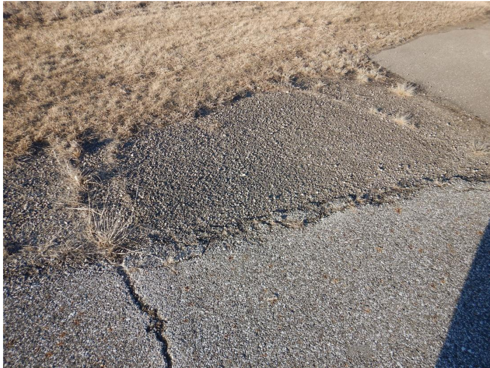
T01FC-02. Raveling (Sample Unit No. 02).
