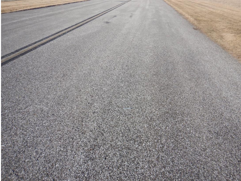
T02FC-01. Bleeding (Sample Unit No. 03) (1).
