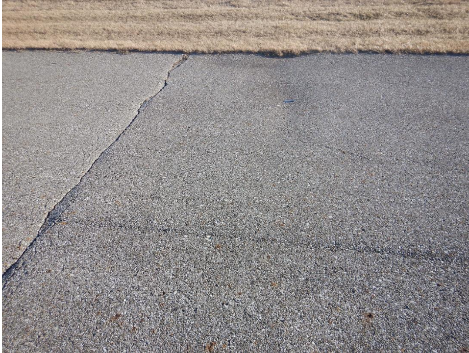
T01FC-02. Depression (Sample Unit No. 01).
