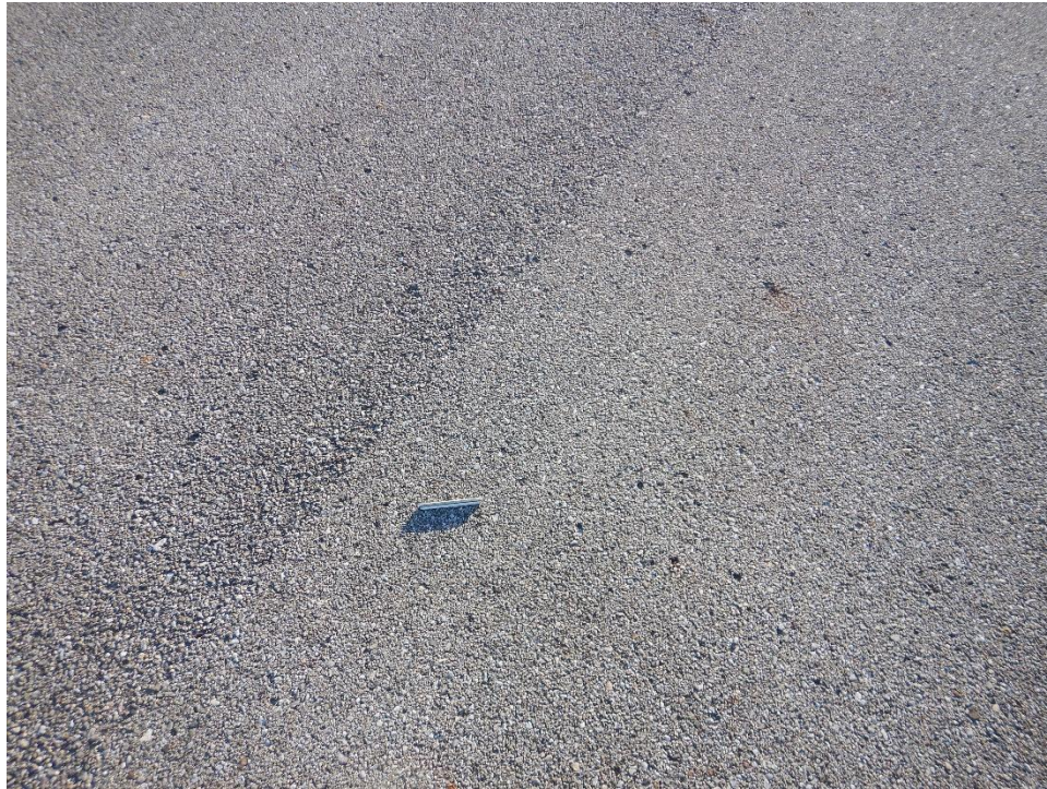
T02FC-02. Weathering (Sample Unit No. 01).
