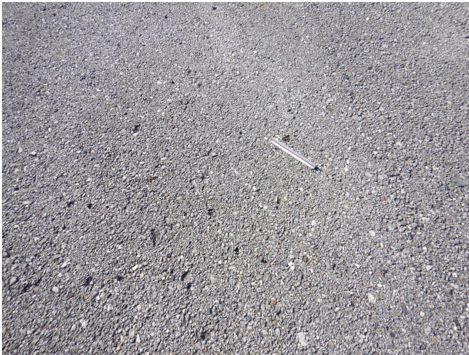
R09FC-04. Raveling (Sample Unit No. 04).
