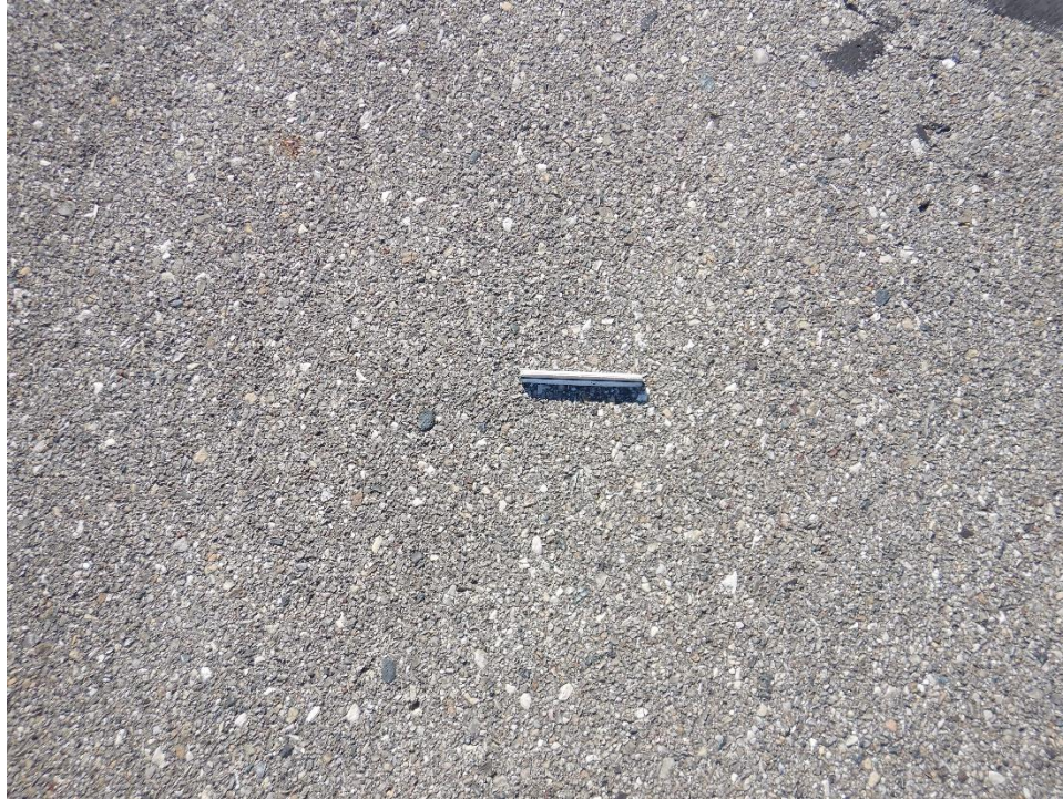
R09FC-03. Weathering (Sample Unit No. 03).
