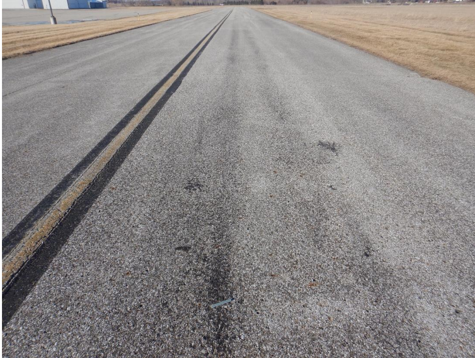
T02FC-01. Bleeding (Sample Unit No. 02) (1).
