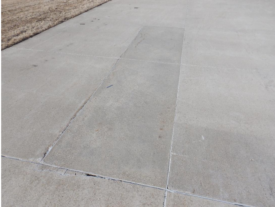
TH01ES-02. Large Patching (Sample Unit No. 02).
