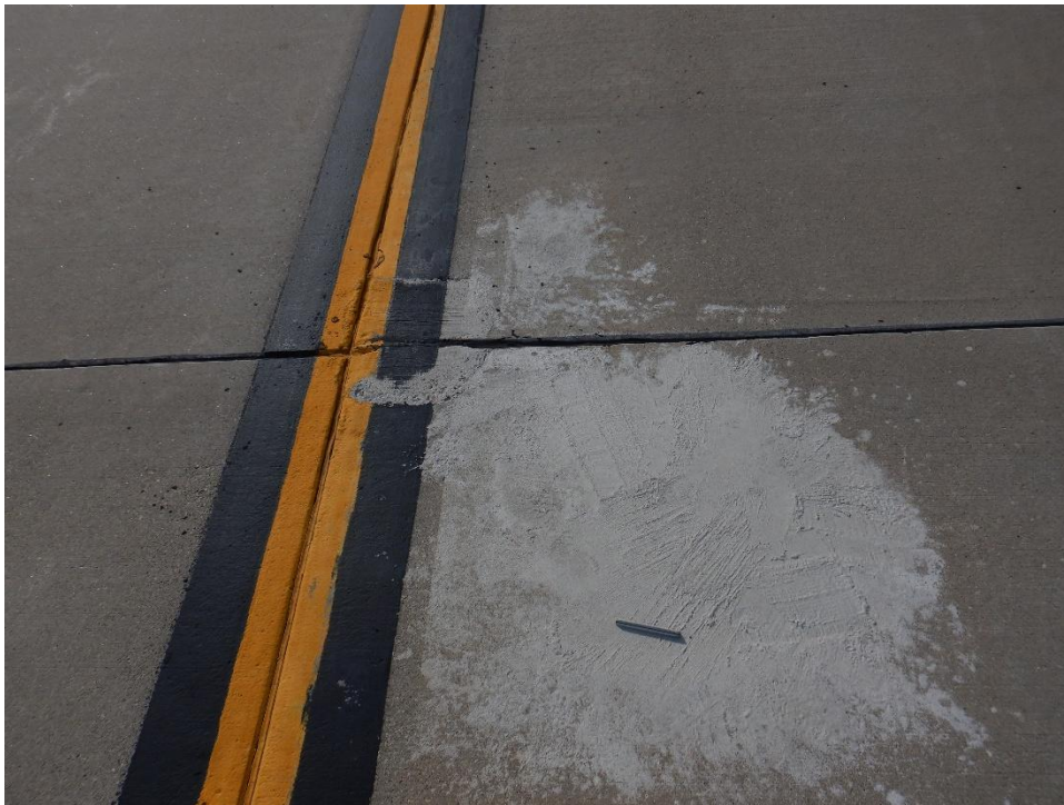
T01ES-01. Small Patching (Sample Unit No. 02).
