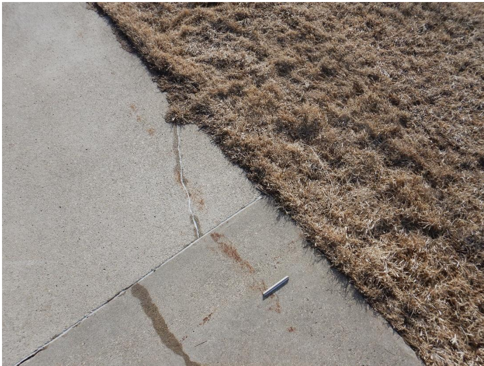
TH01ES-02. Corner Break (Sample Unit No. 02).
