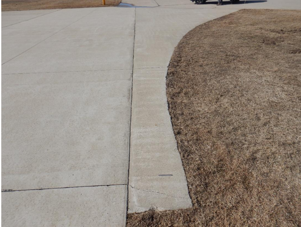
A01EM-02. Corner Break (Sample Unit No. 06).
